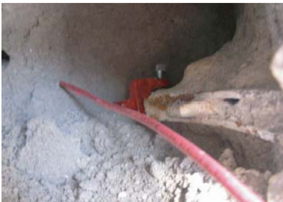
5. C-clamp attached to reinforcement
