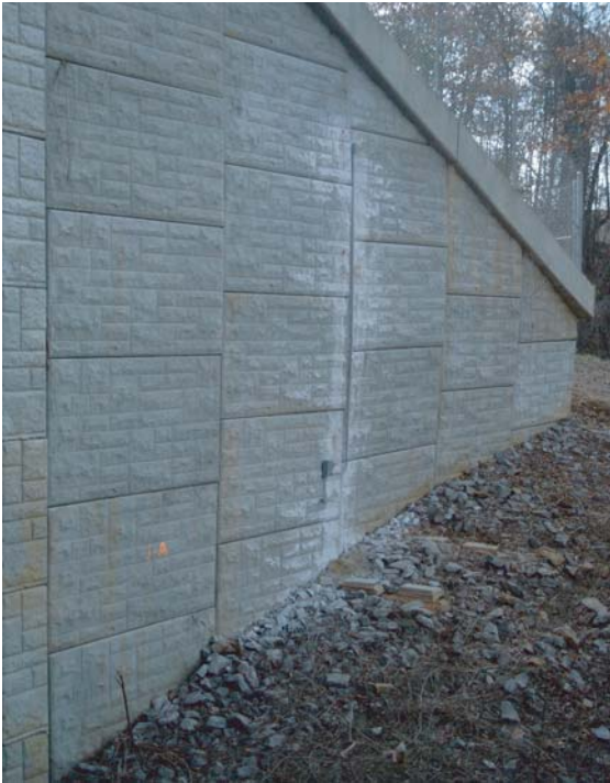
7. Station with junction box
