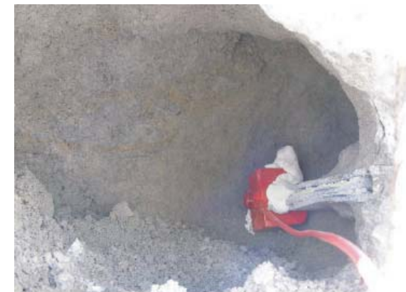
6. C-clamp connection sealed with epoxy
