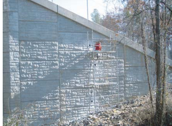
2. Access holes advanced at station
