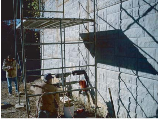
1. Coring hole through precast panel to access backfill and soil reinforcements
