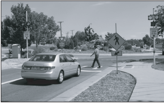
This figure shows a pedestrian-view photograph of the PHB treatment installed at the northwestern approach of the Golden Road two-lane roundabout.
