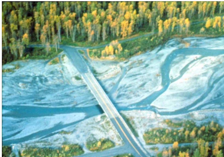
Figure 5-4. Bridge crossing of a braided channel.
