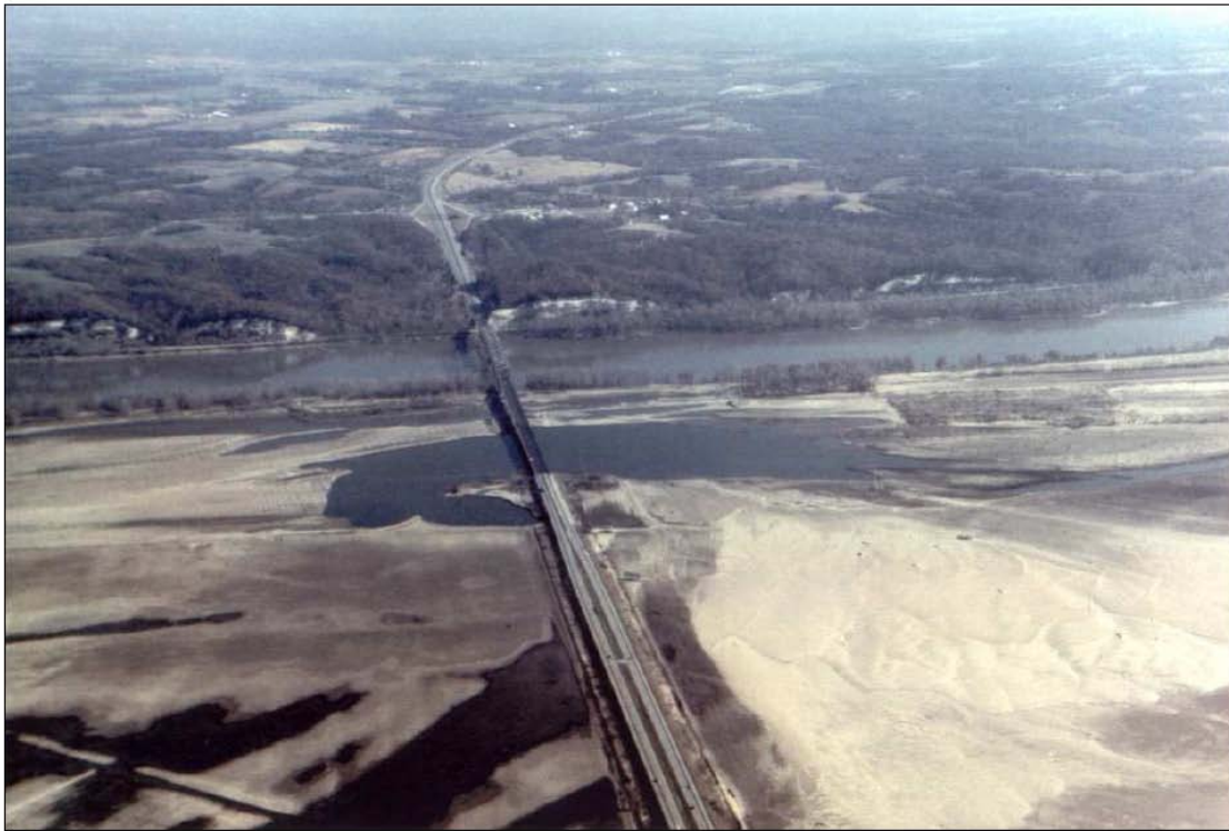
Figure 1-4. Scour at I-70 bridge over Missouri River from 1993 flood. Flow was from left to right. (Photo from Parola et al. 1998).
