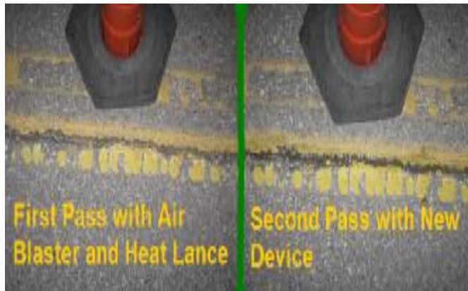
FIGURE 15: A crack after air blasting/heat lance (left) and the same crack after being cleaned by the prototype device (right).
