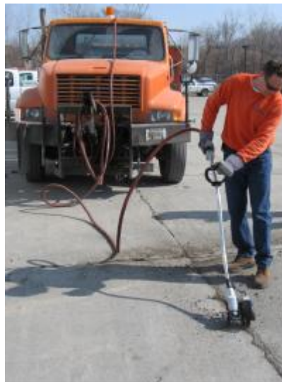
FIGURE 2: Test by a local roads maintenance crew.
