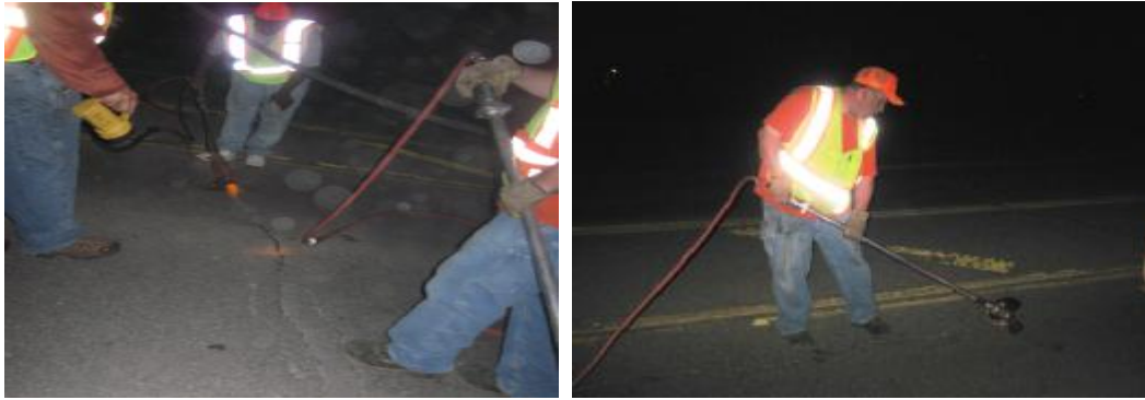
FIGURE 4: NDOR crews using a conventional hot air blaster (left) and the new device (right).
