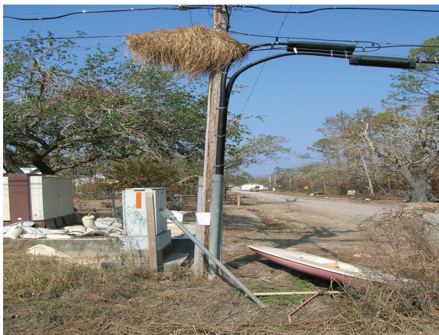
FIGURE 3-4 Sea grass on light pole demonstrates height of the storm surge in a neighborhood adjacent to Bay St. Louis. Source: Hazard and Vulnerability Research Institute, University of South Carolina
