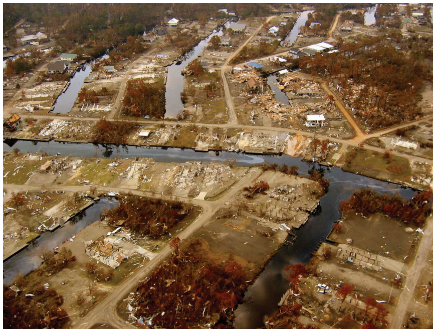
FIGURE 3-5 Many homes in the blocks in the Gulf Coast were destroyed. Source: NOAA ( http://www.katrina.noaa.gov/helicopter/helicopter.html )
