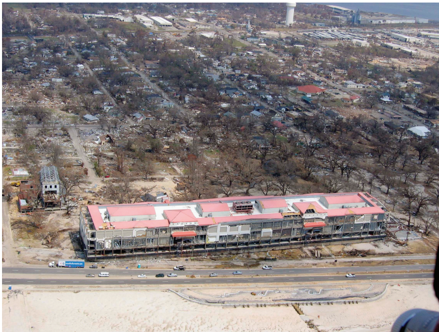
FIGURE 3-6 Part of the Grand Casino Biloxi, which was floating off the beach of Biloxi, was deposited on the other side of the coastal highway by Hurricane Katrina. Source: NOAA ( http://www.katrina.noaa.gov/helicopter/helicopter.html )
