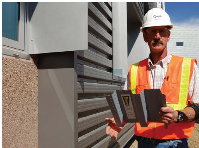
FIGURE G.5 Transpired solar collector. SOURCE: Courtesy of the Department of Energy, National Renewable Energy Laboratory.
