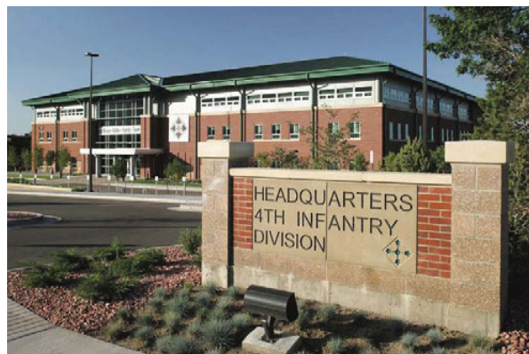
FIGURE E.6 LEED Gold Headquarters of the 4th Infantry Division, Fort Carson, Colorado. SOURCE: Courtesy of the U.S. Army Corps of Engineers.
