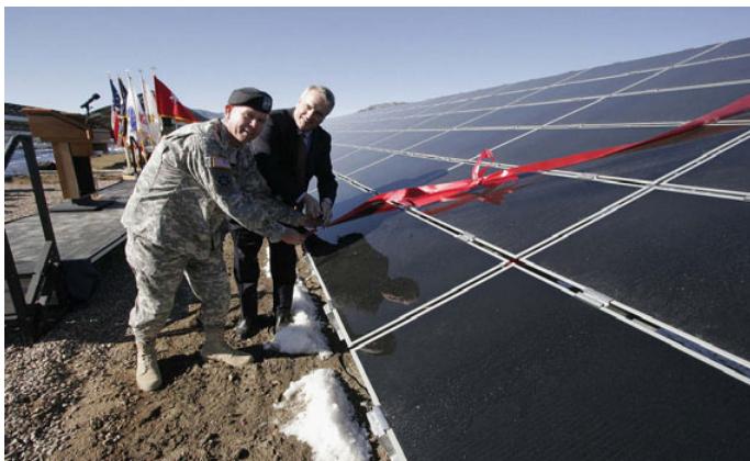
FIGURE E.3 Two-megawatt solar array installed at Fort Carson, Colorado, in 2008. SOURCE: Courtesy of the U.S. Army.
