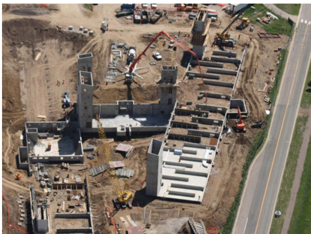
FIGURE G.4 Labyrinth thermal storage at the Research Support Facility. SOURCE: Courtesy of Pat Corkery.
