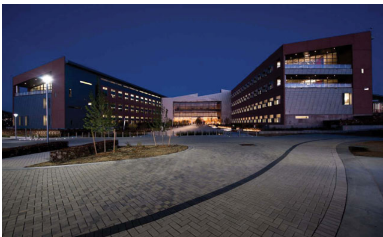
FIGURE G.2 The Department of Energy’s Research Support Facility. SOURCE: Courtesy of the Department of Energy, National Renewable Energy Laboratory.
