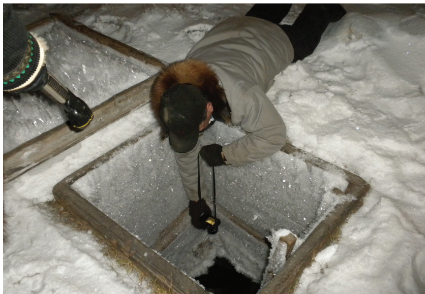
FIGURE 1.5 This photograph is of a cellar in Barrow, Alaska during January 2010. Thawing permafrost can cause damage to infrastructure including ice cellars, which are used in long term storage of traditional foods. Melting can occur during the winter months as well as summer. SOURCE: Michael Brubaker, Alaska Native Tribal Health Consortium.
