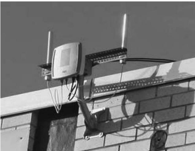
FIGURE 6 Antenna receives wireless data from WMATA buses.
