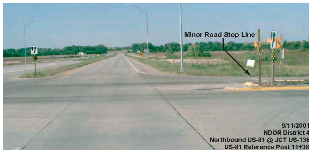
Figure 35. Expressway intersection where minor road stop bar could be moved forward.
