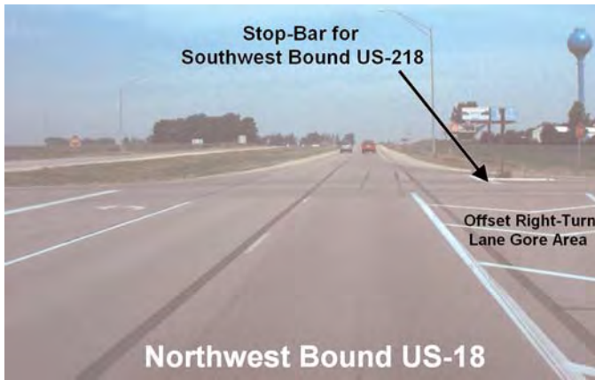
Figure 95. Stop bar location on southwest bound US-218.
