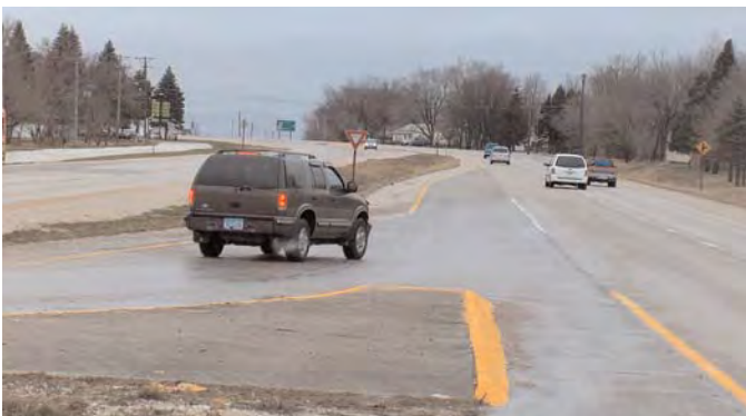
Figure 72. Looking north from south T-intersection at Fort Dodge offset T-configuration.
