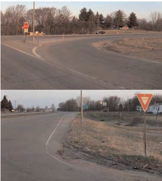
Figure 36. Right-turn acceleration lane in Minnesota.
