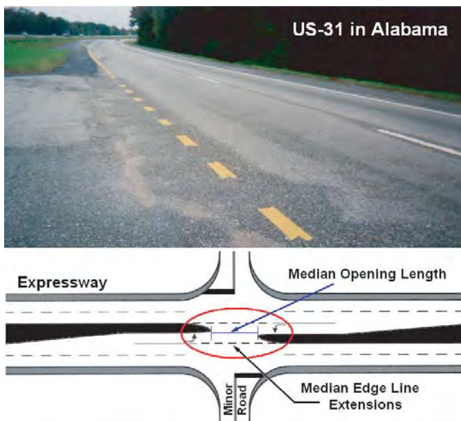
Figure 42. Edge line extensions through median crossover.
