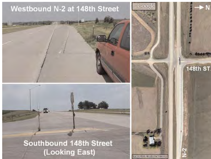
Figure 96. Offset right-turn lane at N-2 and 148th Street near Lincoln, NE.
