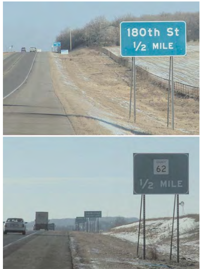
Figure 112. Freeway-style advance intersection guide signing along US-52.
