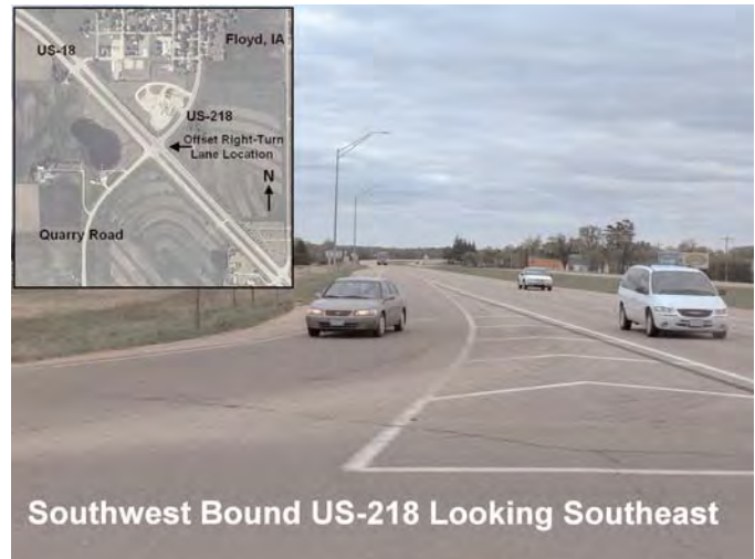
Figure 94. Offset right-turn lane at West Junction of US-18 and US-218, Floyd, IA.
