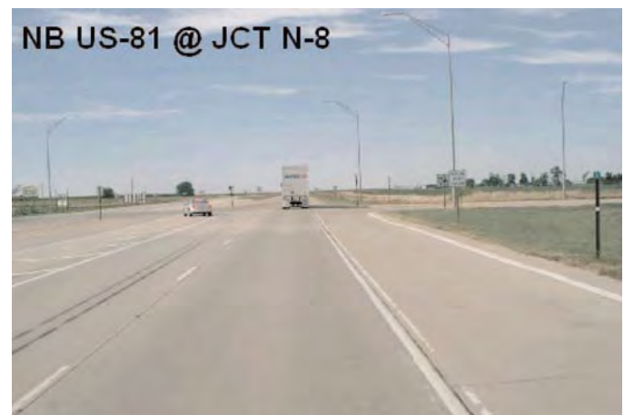
Figure 98. Observed misuse of offset left-turn lane in Nebraska.
