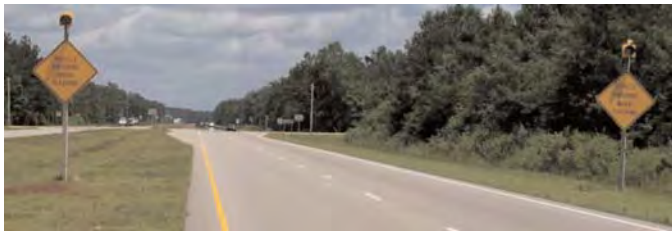
Figure 114. Dynamic VEVF signs on eastbound US-74/76 at SR-1800 (Blacksmith Rd.).
