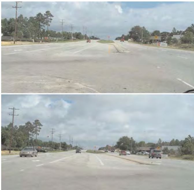
Figure 107. Parallel offset left-turn lanes at US-421 and Golden Road (northbound view) (96).
