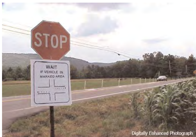
Figure 85. PennDOT static gap assistance treatment application (89).
