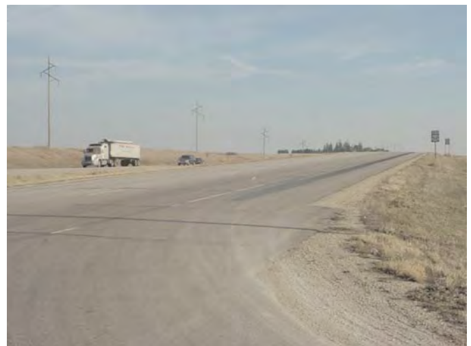
Figure 80. Sight distance issue for eastbound CSAH-9 traffic looking south.
