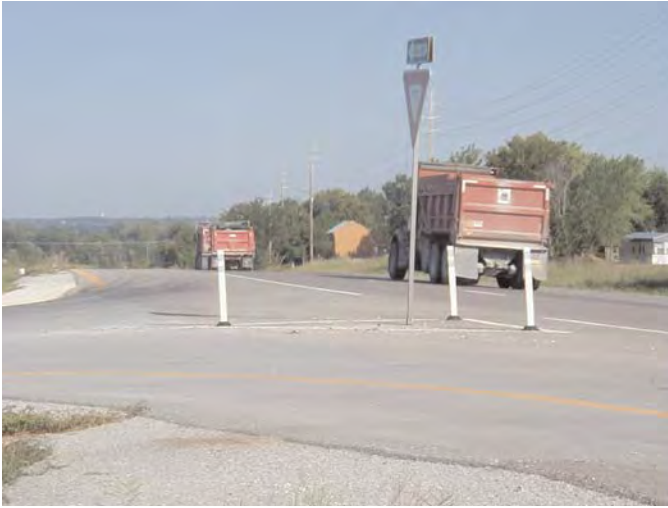
Figure 87. MoDOT MAL with median channelization.
