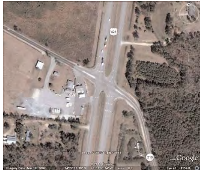
Figure 115. Aerial photo of US-421 and NC-210.
