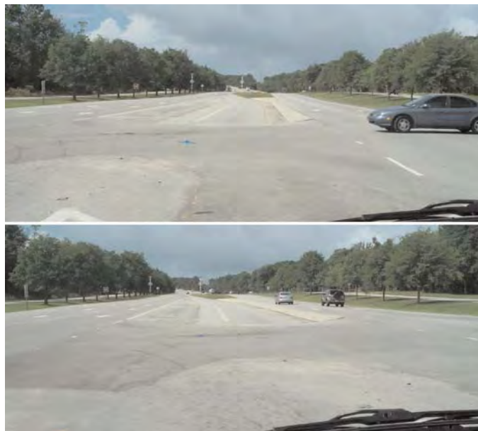
Figure 106. Parallel offset left-turn lanes at US-421 and SR-1576/1531 (southbound view).
