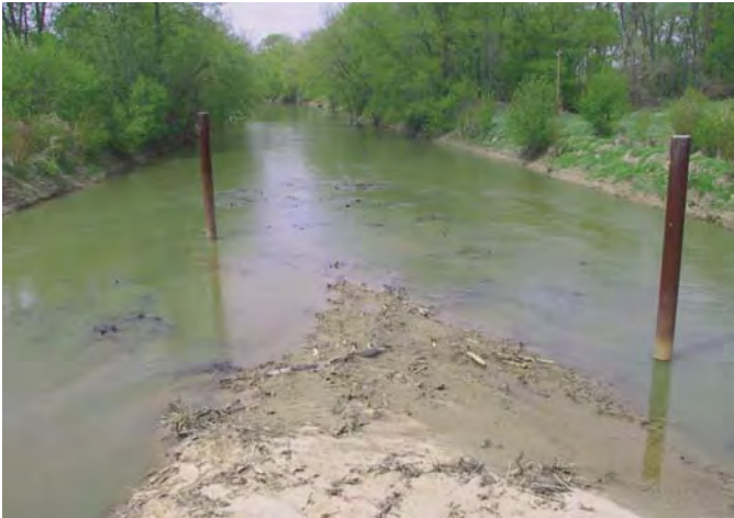
Figure 3.88. Debris deflectors made of steel pipes filled with concrete.
