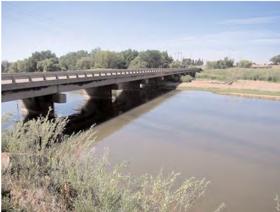
Figure D.4. Looking downstream left bank to right bank at Bridge RD-37.
