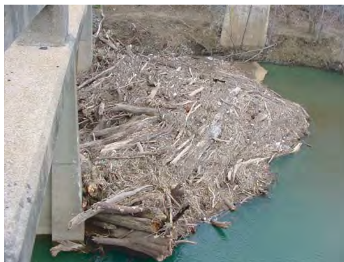
Figure 3.8. View of gap-spanning debris accumulation induced by adjacent pier on the Harpeth River in Tennessee.
