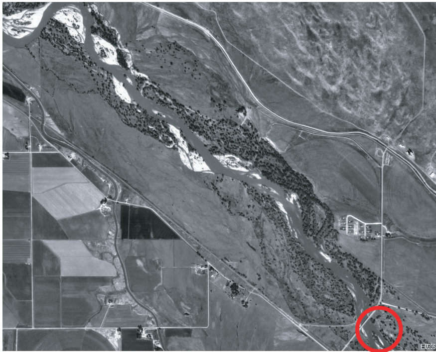
Figure D.13. Aerial view of Bridge RD-50 and the upstream corridor.
