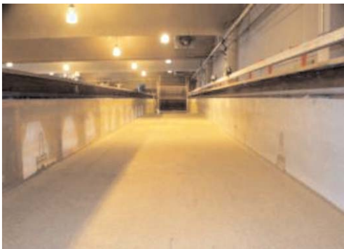
Figure 3.30. Eight-foot (2.4 m) flume before pier installation.
