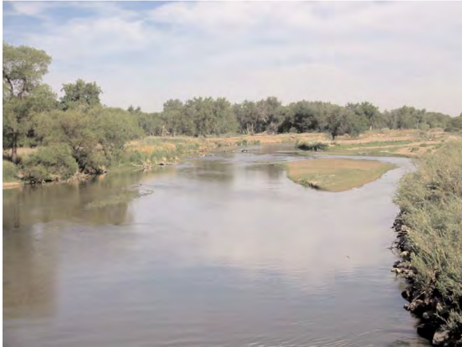
Figure D.6. Looking upstream from Bridge RD-37.
