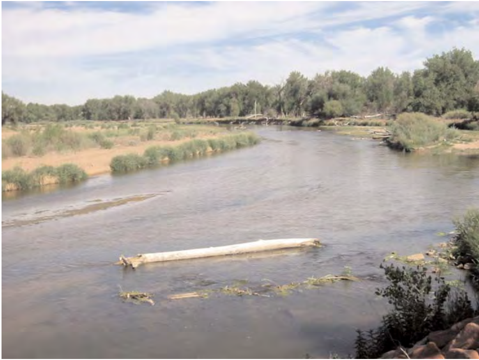
Figure D.14. Looking upstream from Bridge RD-50.
