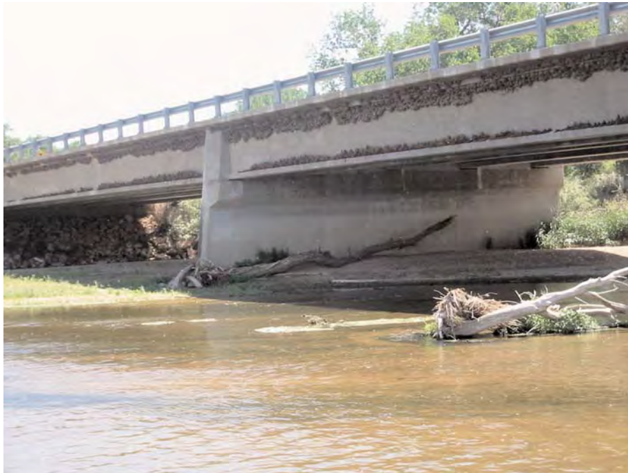
Figure D.8. Left abutment and Pier 1 on Bridge RD-50.
