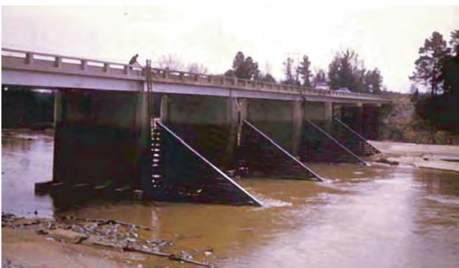
Figure 3.89. Timber debris fins with sloped leading edge.
