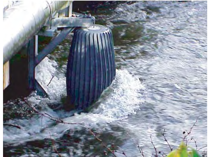
Figure 3.90. Spinning-type debris sweeper.
