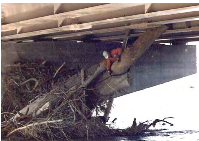
Figure 3.9. View of large debris wedged between bridge substructure and channel bed on Carson River in Nevada.
