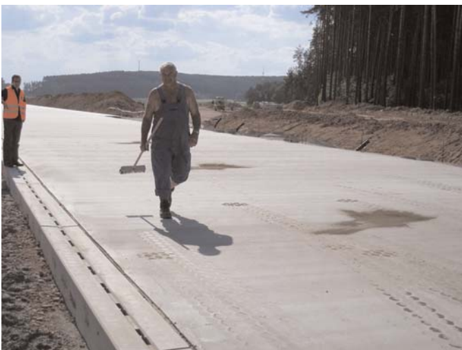
Figure 3.15. Left: Brush operator conducts hand brushing tests at regular intervals to determine when to initiate brushing. Right: First of two passes with brush to develop EAC texture.
