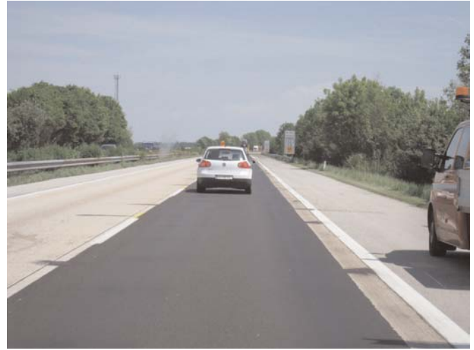
Figure 3.41. The old two-layer PCC Regau section, built in the 1960s, has a thin asphalt surface placed on the driving lane. The passing lane has the original concrete surface, which is more than 42 years old.
