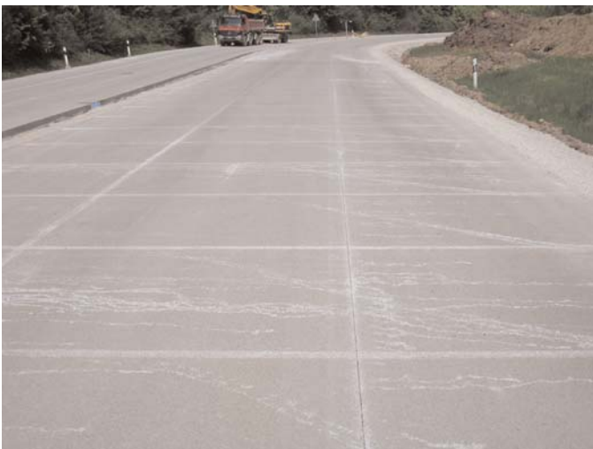
Figure 3.36. Left: Finished whitetopped ramp along A99. Right: A handful of polypropylene fibers included in PCC for the A99 project.
