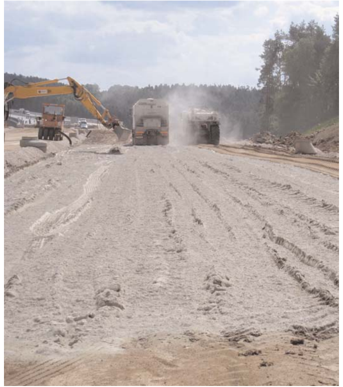
Figure 3.5. Left: Site cleared for two lanes in each direction. Right: Stabilizing the subgrade with cementitious compound.
