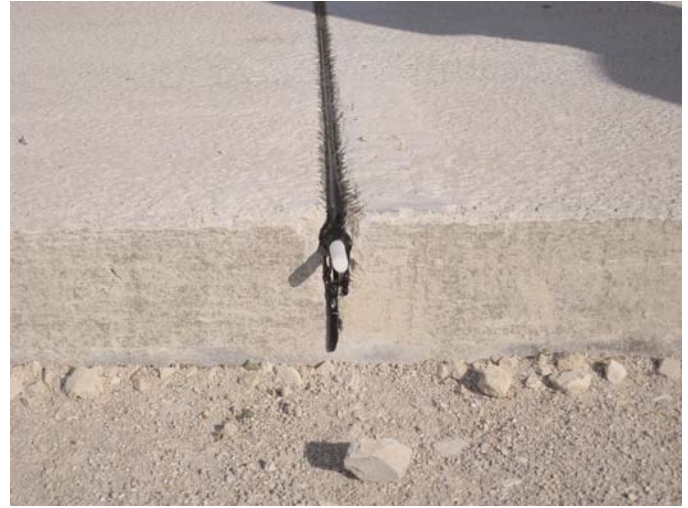
Figure 3.19. Left: Finished two-layer EAC pavement. Right: Bituminous seal used for both longitudinal and transverse joints.
