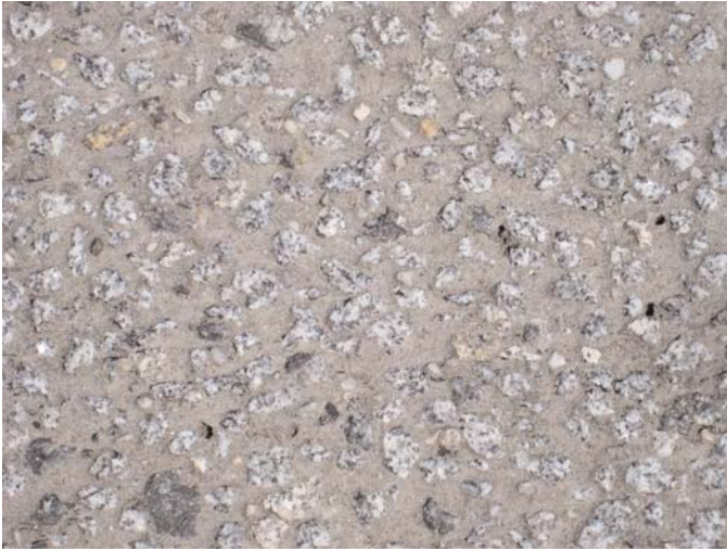
Figure 3.35. Texture close-ups in EAC sections and close-up of bituminous seal used on both transverse and longitudinal joints on A93 Section P (km 12.500–22.780).
