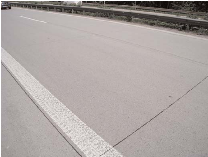
Figure 3.34. Top: SMA over PCC in Section N (km 8.600–11.000). Bottom: Sections similar to Section N were reclaimed for EAC/PCC in new Section P (km 12.500–22.780).
