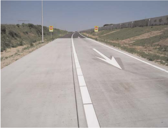
Figure 4.10. A ramp end on the A73 showing the unsurfaced CRCP.
