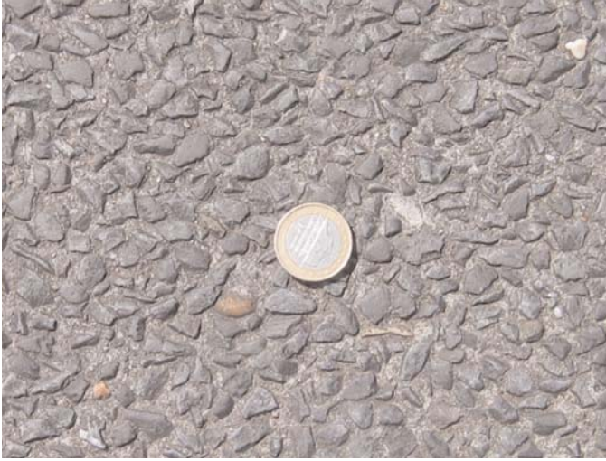
Figure 3.28. Texturing on a 5/8-mm section along N279 in the Netherlands.
