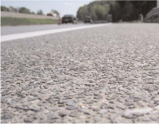
Figure 3.39. The exposed aggregate texturing on the Eugendorf section.
