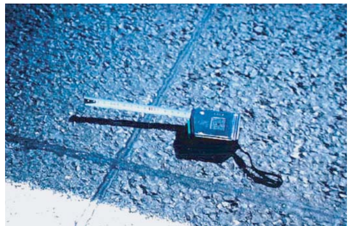
Figure 4.12. Sawed and sealed joints on the A11 near Berlin in 1993 (5).
