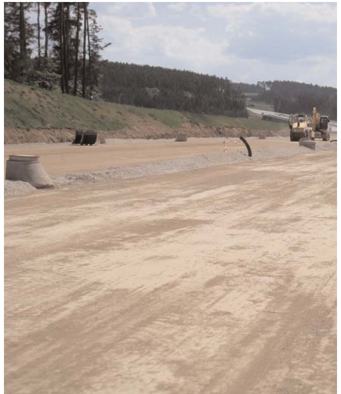
Figure 3.6. Left: Frequent spraying of base layer in front of the first paver minimizes moisture loss in the lower layer of PCC to base. Right: Prepared, stabilized subgrade awaits frost blanket aggregate layer.
