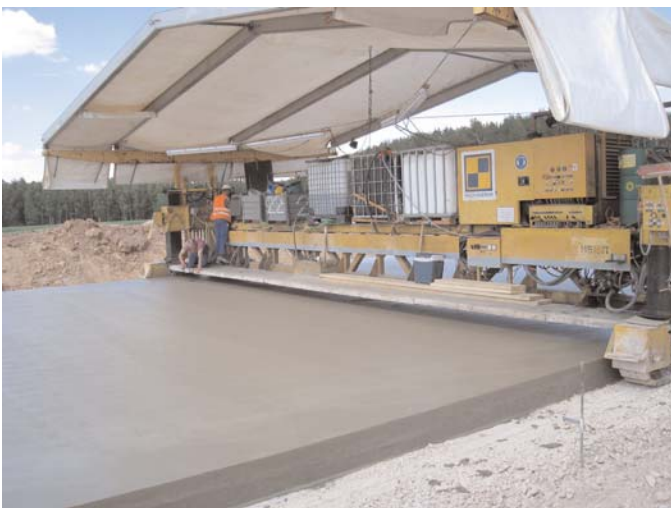
Figure 3.11. Left: Front view of the final machine in the paving train, the finishing machine. Right: A close-up of last-second touch-ups as the finishing machine continues along.
