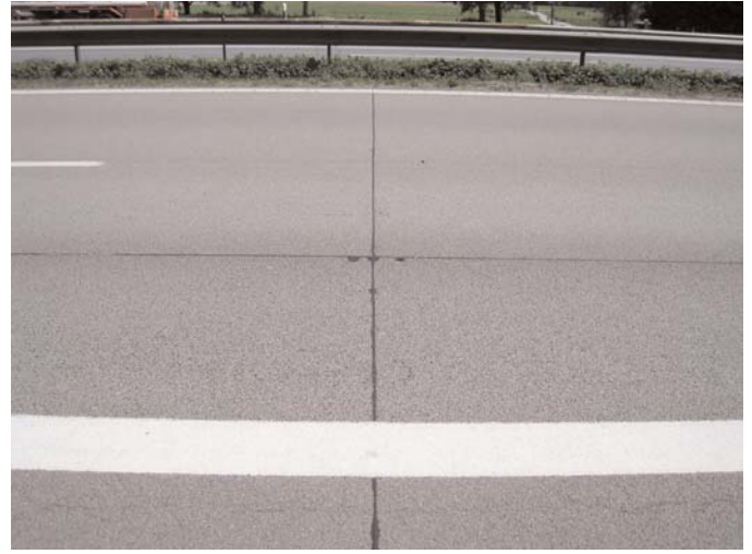
Figure 4.17. A93 motorway showing transverse sawed and sealed joint in SMA over JPCP after 13 years of heavy traffic. In center of photo, note longitudinal joint that is also sawed and sealed.
