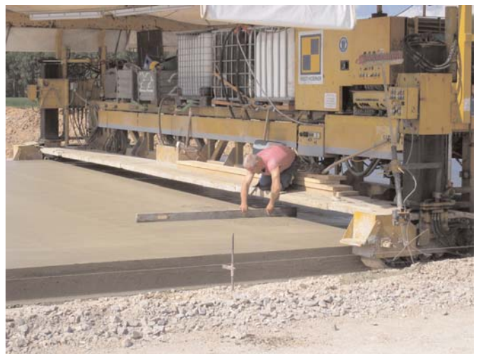
Figure 3.11. Left: Front view of the final machine in the paving train, the finishing machine. Right: A close-up of last-second touch-ups as the finishing machine continues along.
