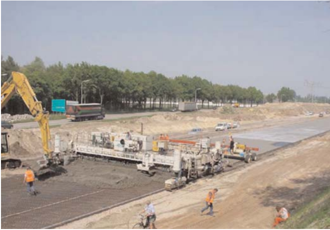
Figure 4.8. Paving of CRCP motorway in the Netherlands.
