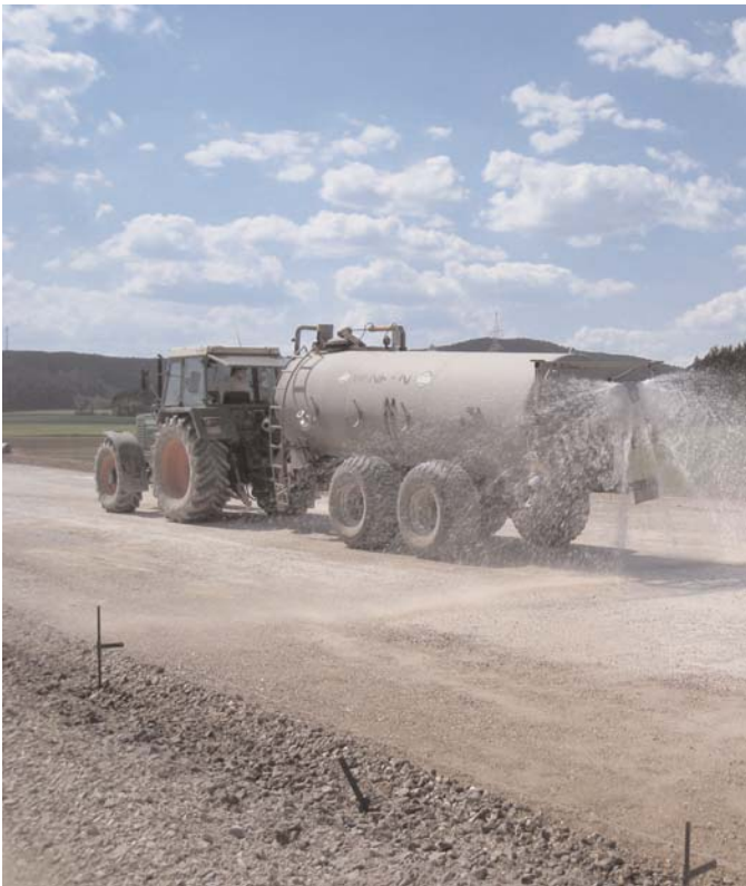
Figure 3.6. Left: Frequent spraying of base layer in front of the first paver minimizes moisture loss in the lower layer of PCC to base. Right: Prepared, stabilized subgrade awaits frost blanket aggregate layer.
