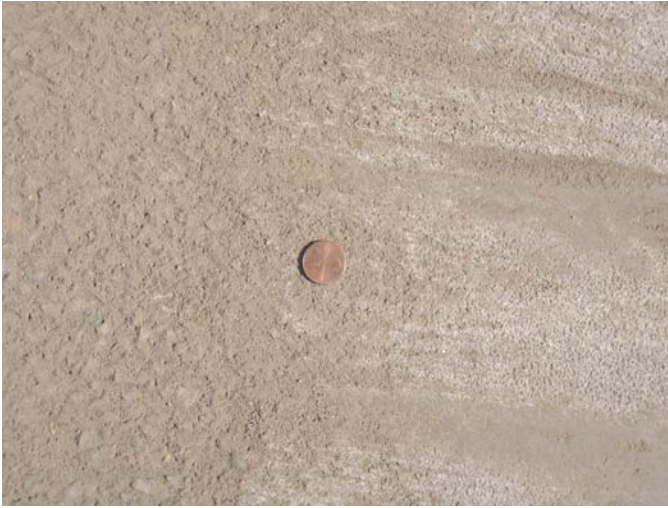
Figure 3.16. EAC texture after first pass of brush is shown in left half of photo. Unbrushed surface with compound still visible is shown in right half of photo.
