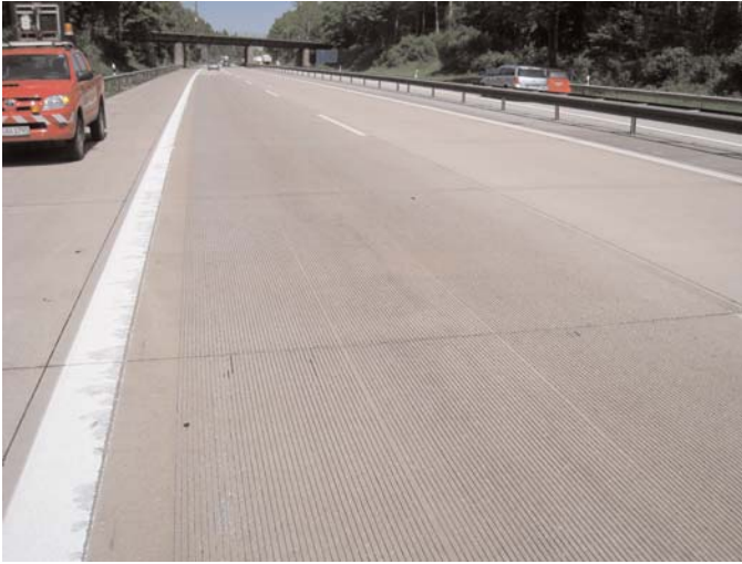
Figure 3.32. Left: Grooved texture on section along A93 (km 5.600–5.700). Right: Diamond-ground texture on another section of A93 (km 5.900–5.950).
