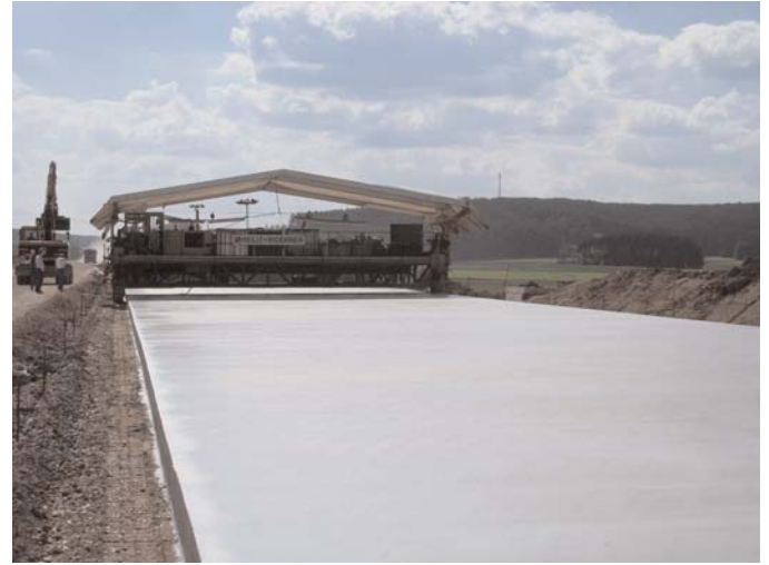
Figure 3.12. Left: Rear view of the finishing machine with spray arm attachment. Right: View of placed two-layer PCC slab with combination curing compound and retardant sprayed on surface.
