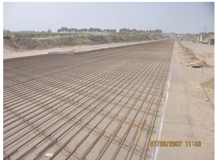
Figure 4.7. A73 CRCP reinforcing steel. The transverse supports are placed at a 20-degree angle from transverse perpendicular.
