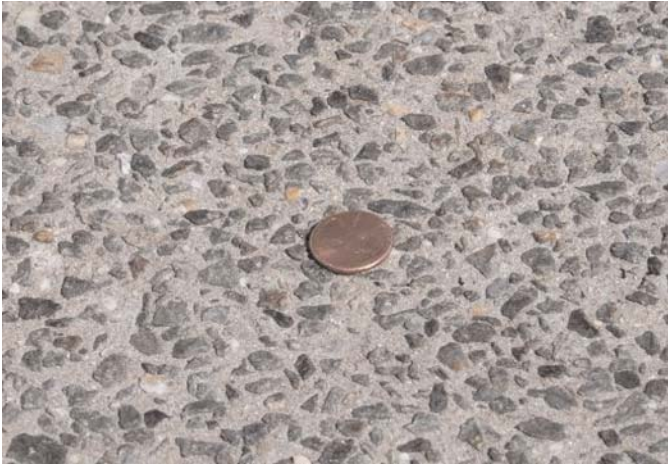
Figure 3.1. An example of exposed aggregate texture (with maximum aggregate size of 8 mm) of a two-layer PCC pavement taken along the A1 motorway near Eugendorf, Austria.
