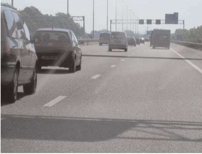
Figure 4.4. A12 motorway between Utrecht and Ede after 10 years in service.
