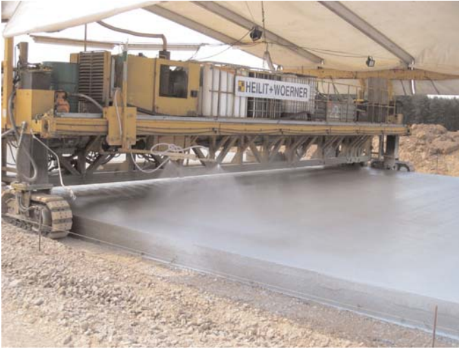
Figure 3.12. Left: Rear view of the finishing machine with spray arm attachment. Right: View of placed two-layer PCC slab with combination curing compound and retardant sprayed on surface.
