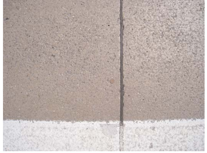
Figure 3.30. Significant polishing of burlap drag after 13 years of traffic on A93, Section A (km 1.490–1.910).
