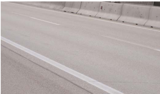
Figure 3.43. The Vorchdorf sections showed noticeable polishing in the wheelpaths despite being only 9 years old.
