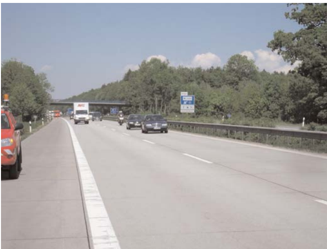
Figure 3.33. Exposed aggregate section and texture (km 7.440–8.600).
