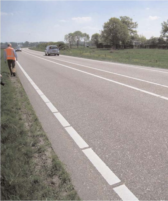
Figure 3.25. The 4/22-mm sections along N279 in the Netherlands.
