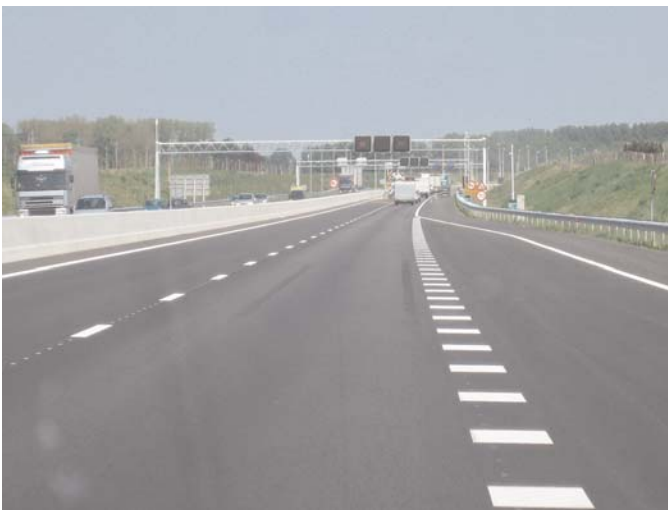
Figure 4.5. Completed A73 composite AC/CRCP motorway in the Netherlands, May 2008.
