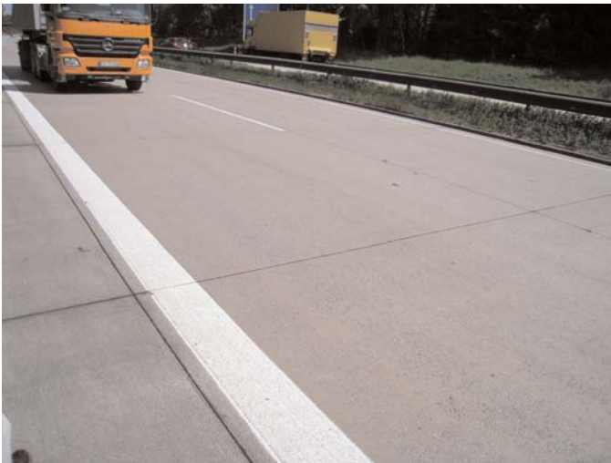
Figure 3.29. Original burlap drag on A93, Section A (km 1.490–1.910).
