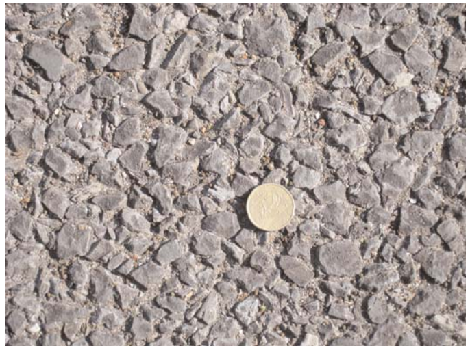
Figure 4.3. Close-up of the porous asphalt surface of the A12 motorway. Note fines infiltrating the porous asphalt surface on the edge of the traffic lane.
