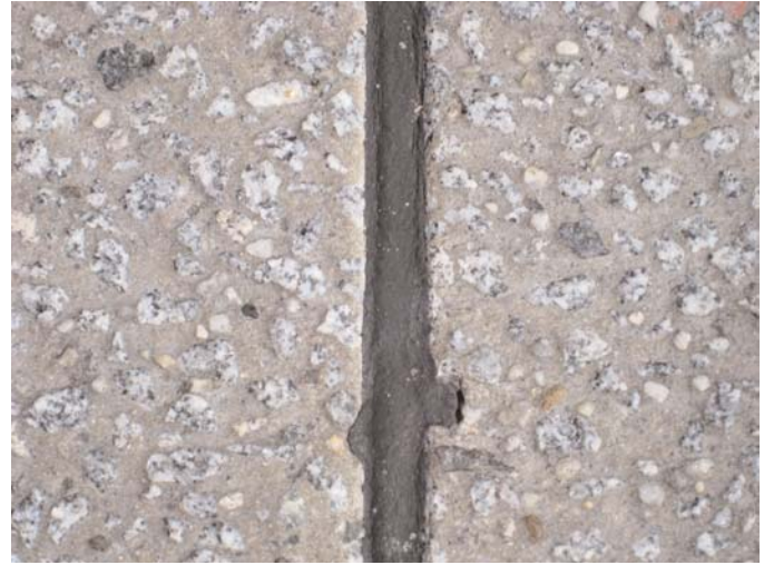
Figure 3.35. Texture close-ups in EAC sections and close-up of bituminous seal used on both transverse and longitudinal joints on A93 Section P (km 12.500–22.780).
