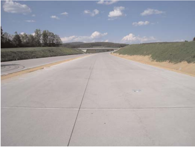
Figure 3.19. Left: Finished two-layer EAC pavement. Right: Bituminous seal used for both longitudinal and transverse joints.
