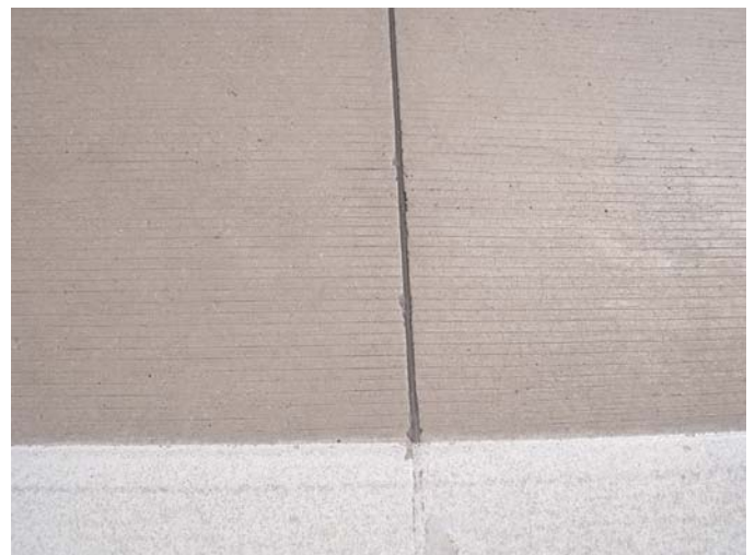
Figure 3.31. Top: Longitudinal tining known as “American comb” (km 1.910–2.070). Bottom: “Spanish comb” (km 2.070–3.335).
