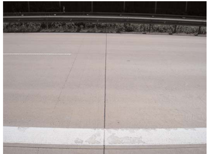
Figure 3.30. Significant polishing of burlap drag after 13 years of traffic on A93, Section A (km 1.490–1.910).
