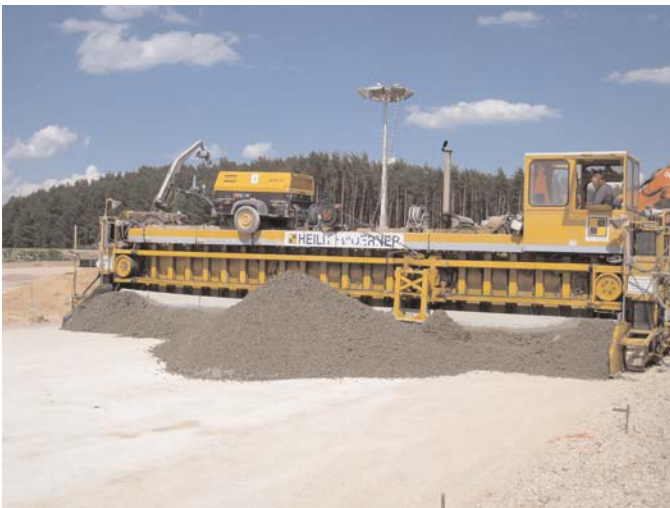
Figure 3.8. Close-up of the rear of the first paving machine, which has an automated dowel inserter attachment. Inset: A tiebar and a dowel.
