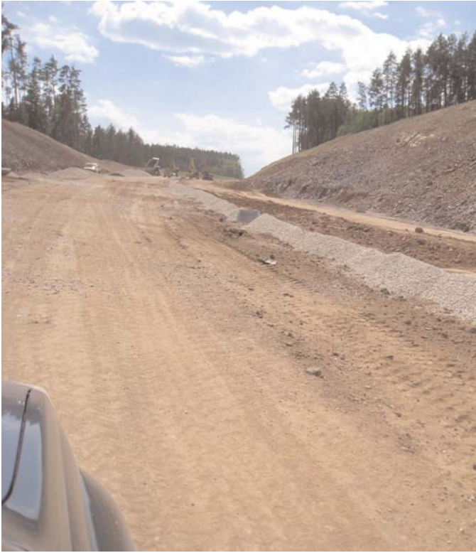
Figure 3.5. Left: Site cleared for two lanes in each direction. Right: Stabilizing the subgrade with cementitious compound.
