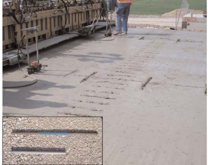
Figure 3.8. Close-up of the rear of the first paving machine, which has an automated dowel inserter attachment. Inset: A tiebar and a dowel.
