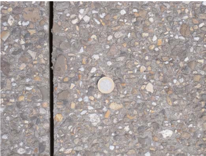
Figure 3.26. The texturing on the 4/22-mm sections along N279 in the Netherlands.
