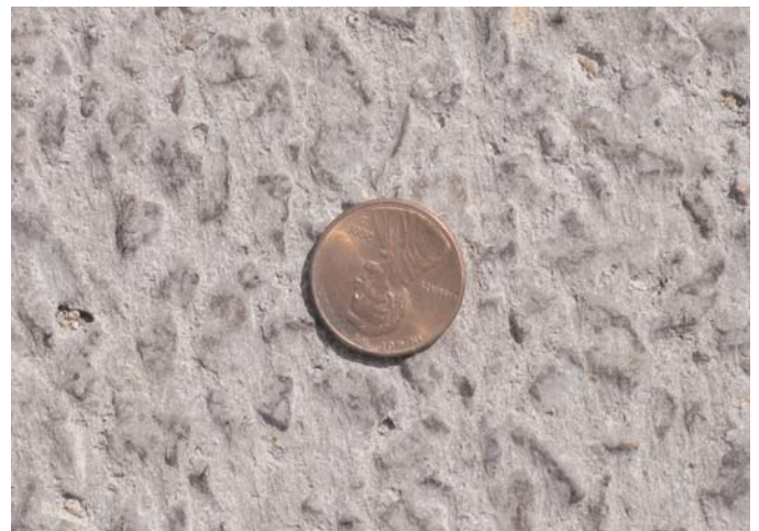
Figure 3.18. Close-up of finished EAC texture on sections constructed on A6.
