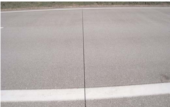
Figure 3.40. The section at Eugendorf exhibited slight wear in the wheelpaths of the driving lane, resulting mainly from 14 years of regular salting and plowing and 10 years of studded tires.
