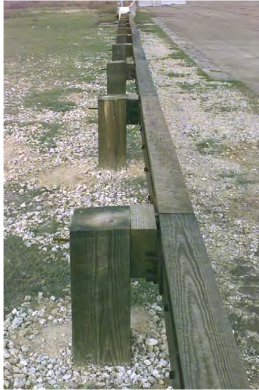
Figure 9. Type A Steel-Backed Timber Guardrail System.
