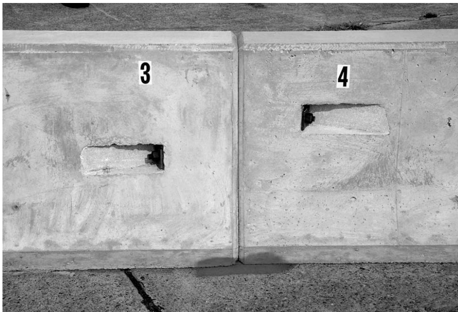
Figure 21. F-Shape Concrete Safety Barrier with X-Bolt Connection.
