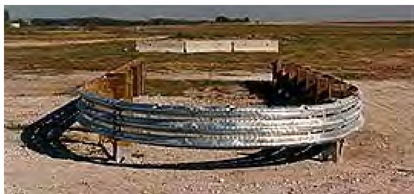
Figure 31. Bullnose Attenuator.
