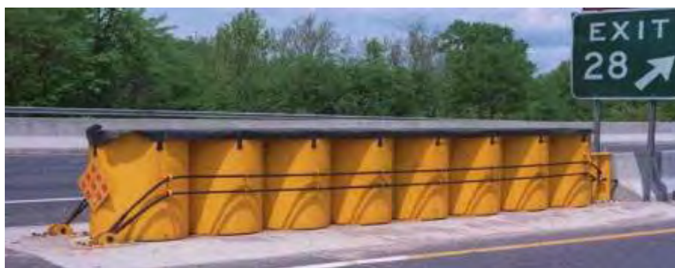
Figure 30. Narrow Connecticut Impact Attenuator System.
