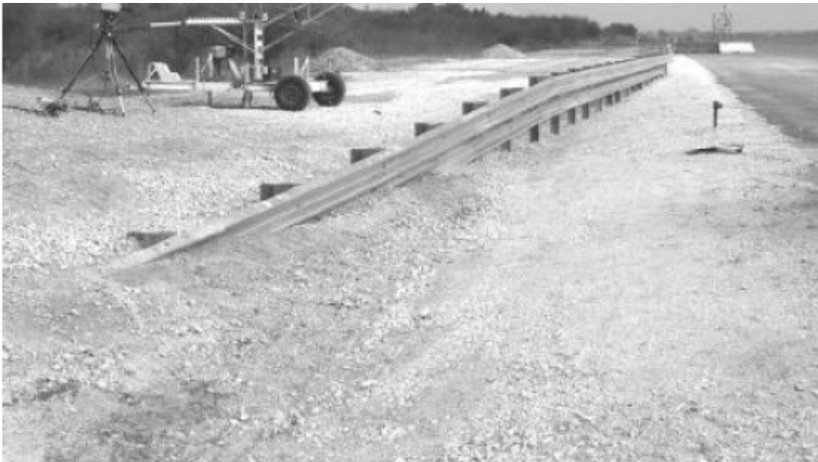
Figure 24. Buried-in-Backslope Guardrail Terminal.
