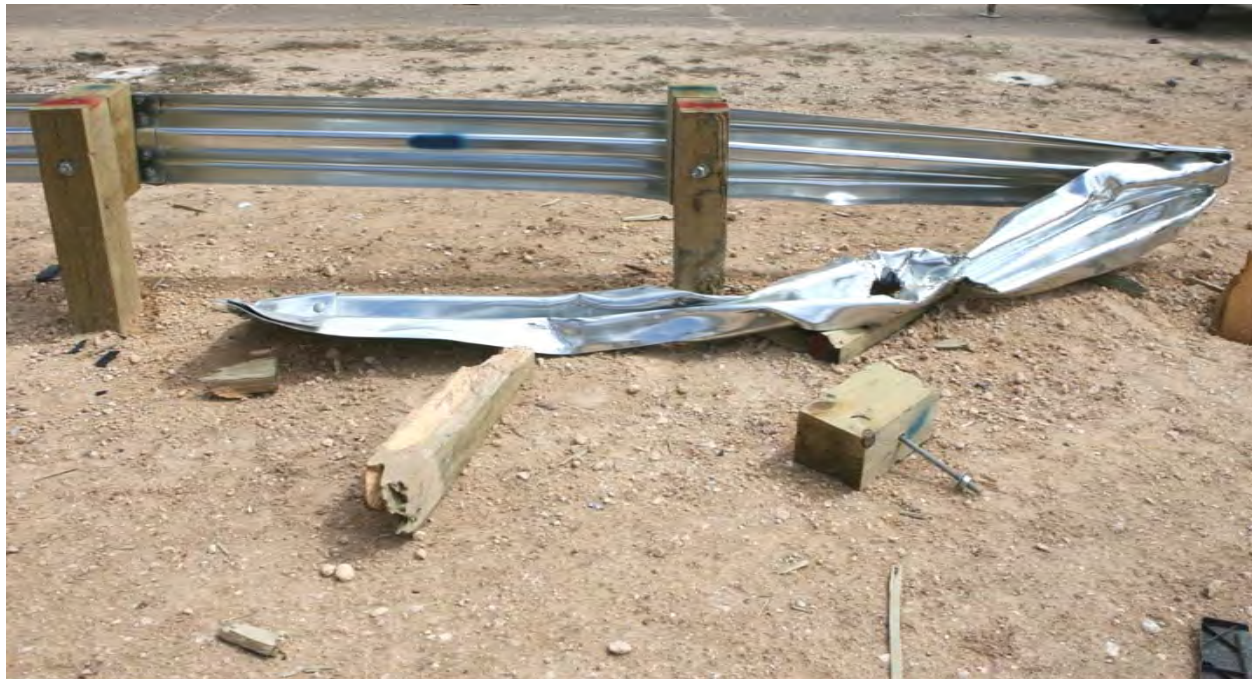
Figure 48. G4(2W) W-Beam Guardrail after MASH Test 3-11.
