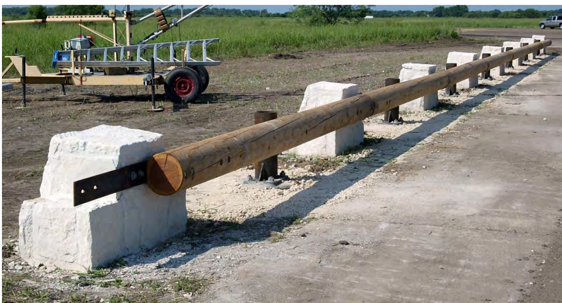
Figure 13. Deception Pass State Park Log Rail System.
