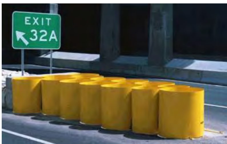
Figure 29. Connecticut Impact Attenuator System.
