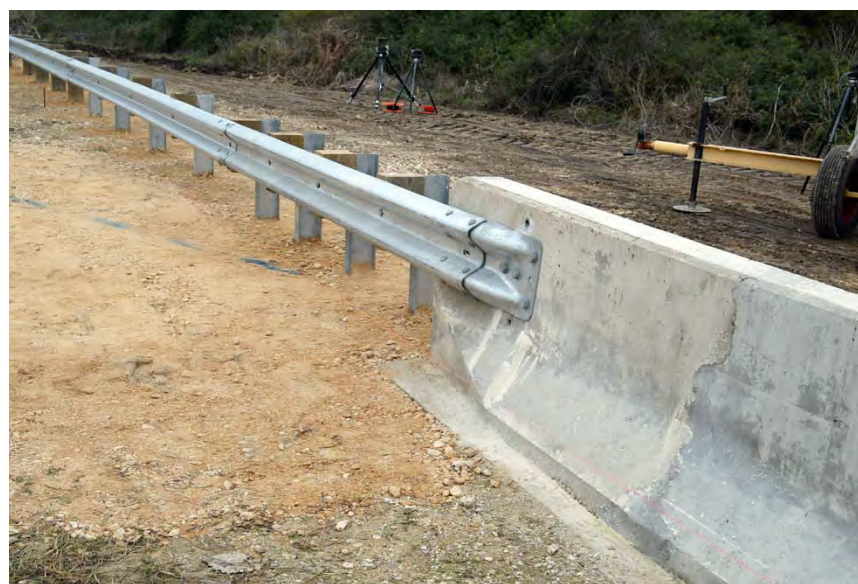
Figure 23. Texas TL-2 Guardrail-to-Concrete Bridge Rail Transition.
