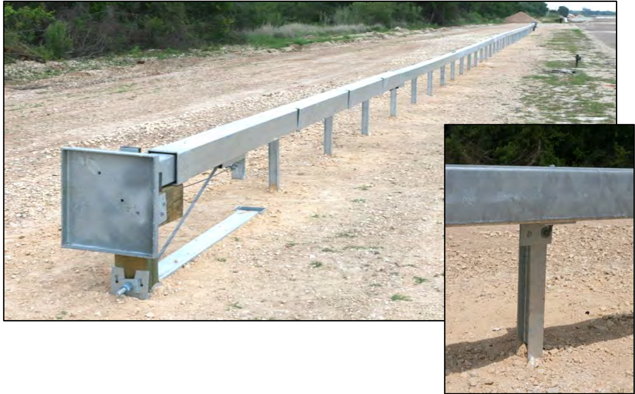
Figure 73. G3 Weak Post Box-Beam Guardrail prior to Testing.
