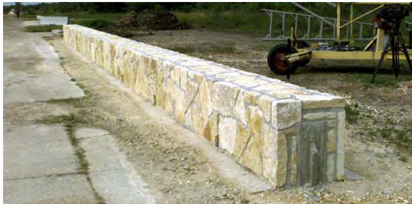
Figure 8. Rough Stone Masonry Guardwall System.
