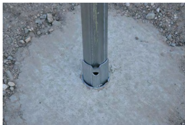
Figure 33. Photographs of Wedge Anchor Sign Support.
