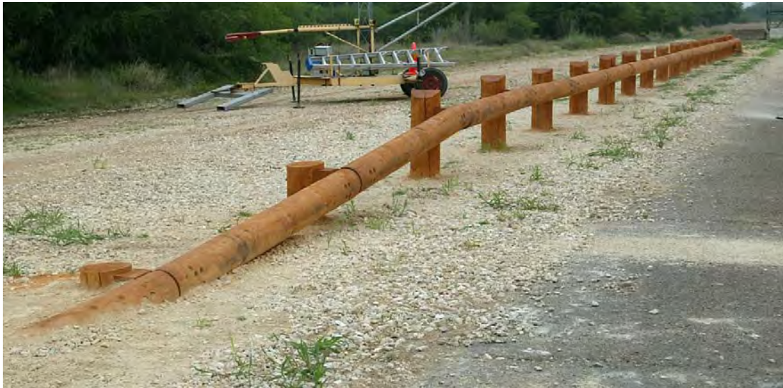
Figure 12. Round Steel-Backed Timber Guardrail System.
