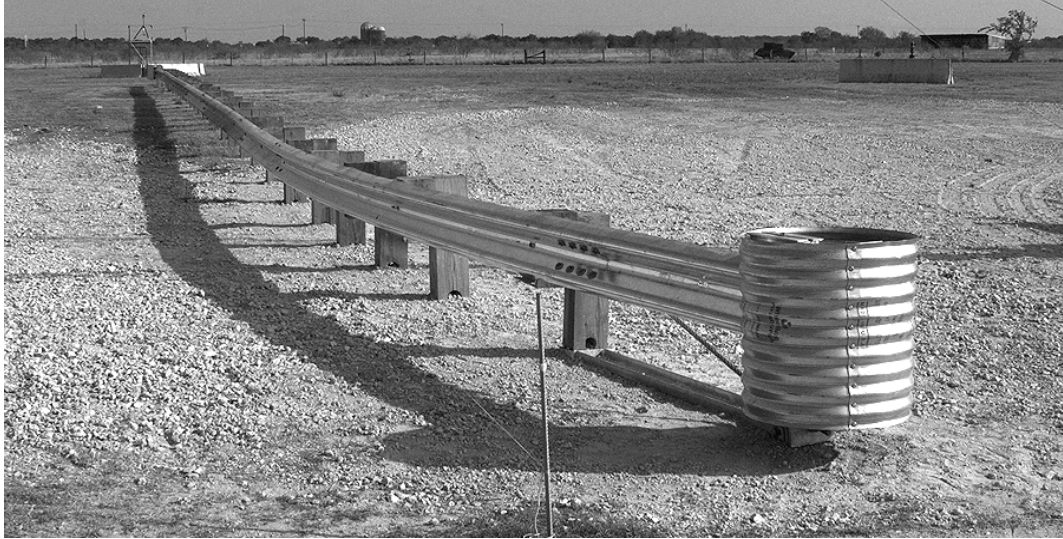
Figure 25. Eccentric Loader Terminal.
