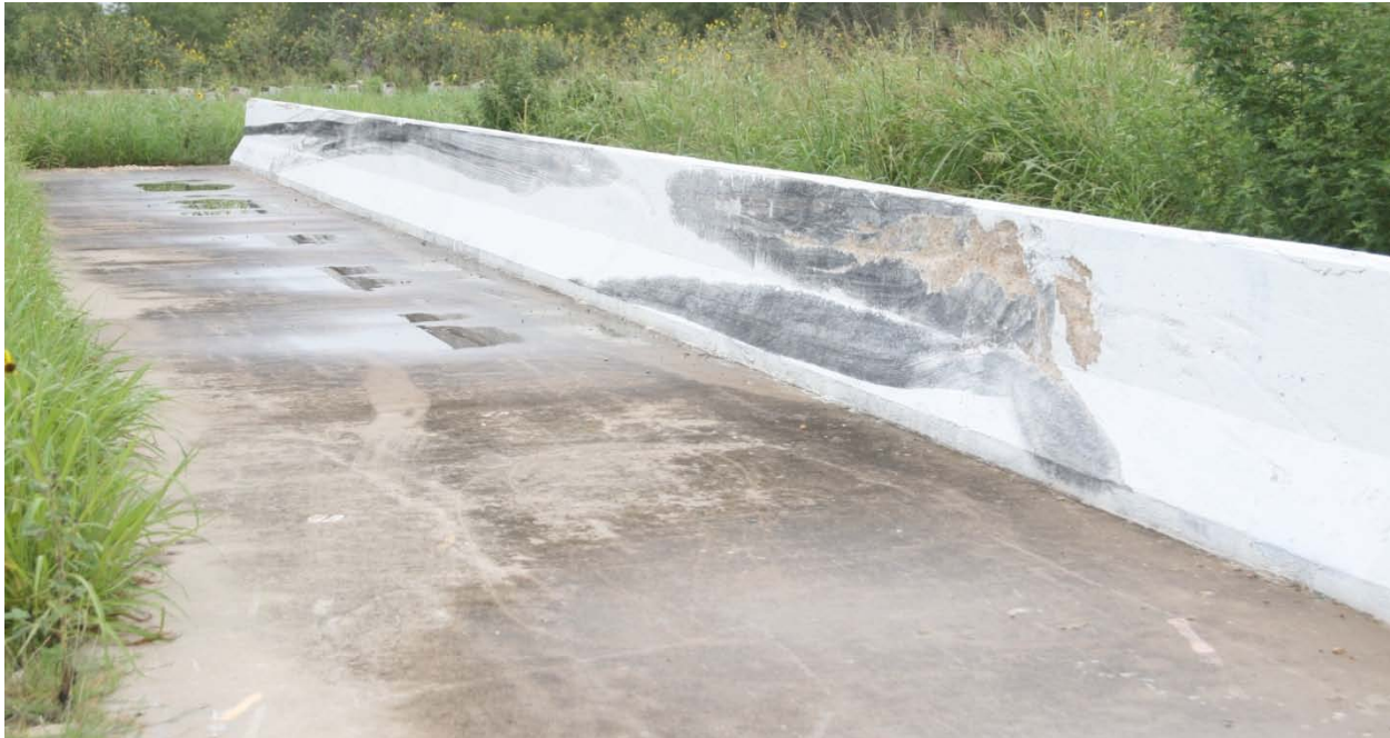
Figure 40. 32-inch New Jersey Shape Barrier after MASH Test 4-12.
