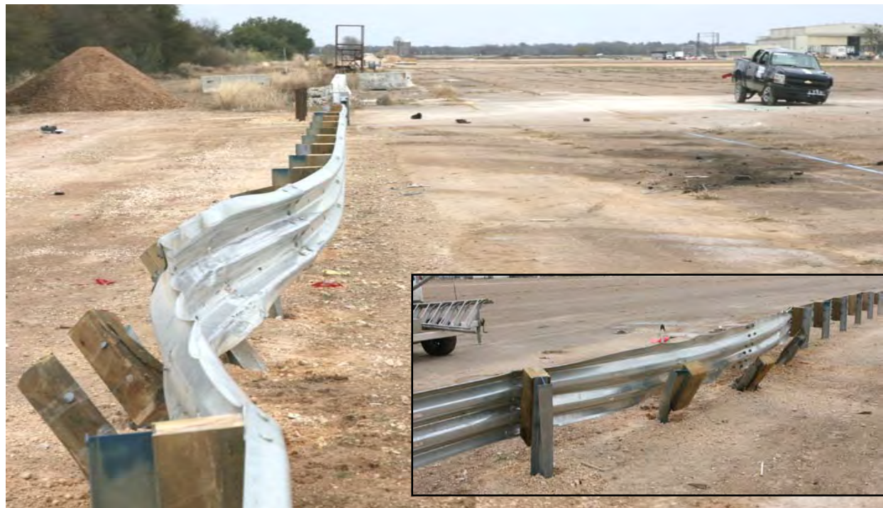
Figure 84. G9 Thrie Beam Guardrail after MASH Test 3-11.
