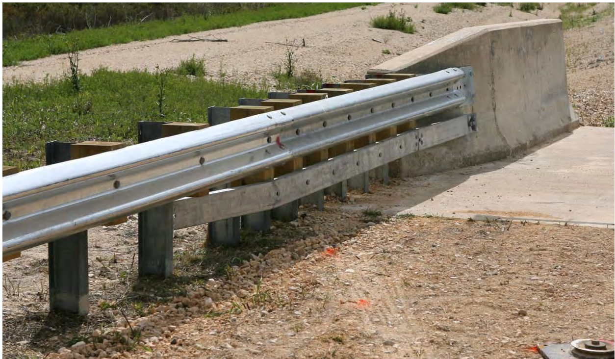
Figure 60. W-Beam Transition prior to Testing.
