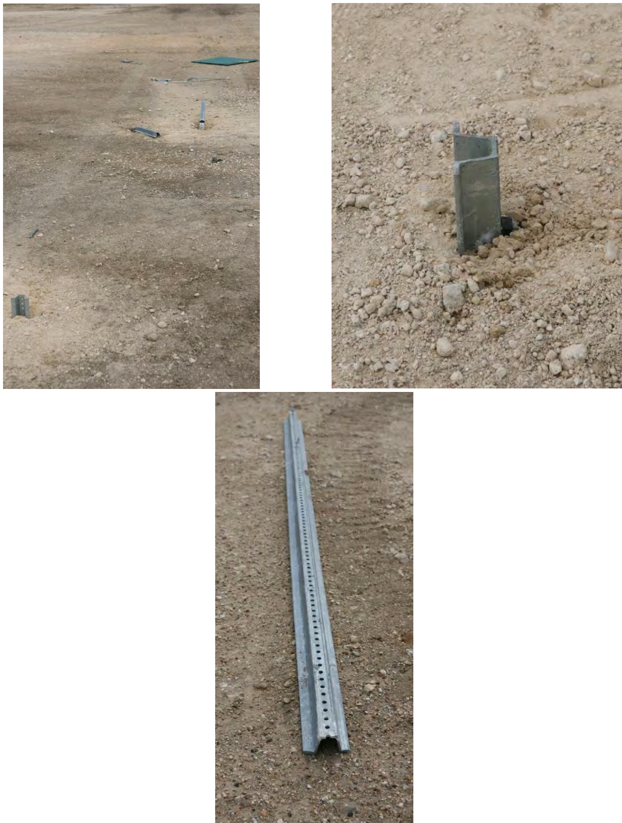
Figure 68. U-Channel Installation after MASH Test 3-62.
