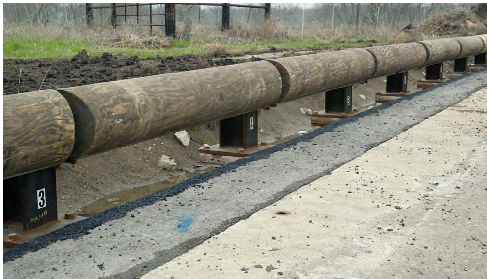
Figure 15. Glacier Park Round Removable Timber Guardrail System.
