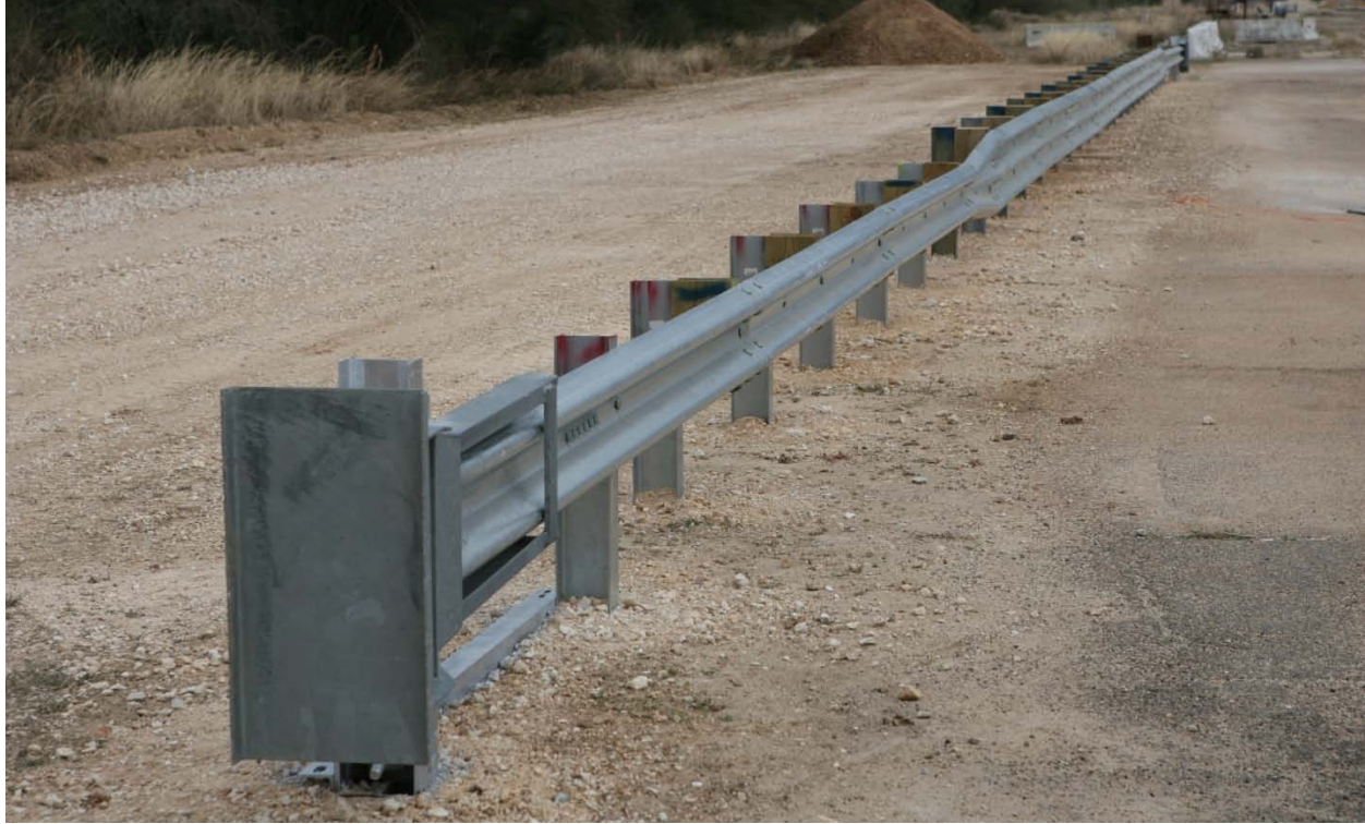
Figure 83. G9 Thrie Beam Guardrail prior to Testing.
