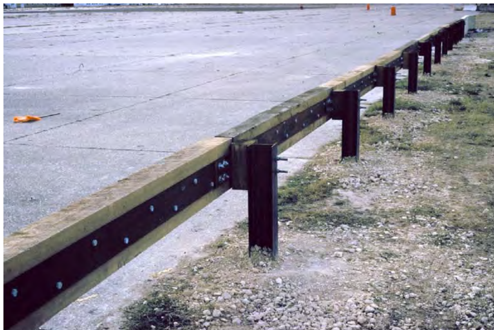
Figure 10. Merritt Parkway Steel-Backed Timber Guardrail System.
