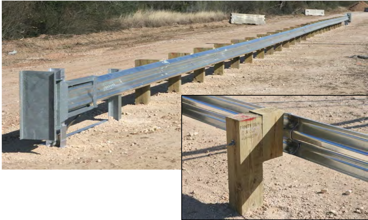
Figure 47. G4(2W) W-Beam Guardrail Prior to Testing.
