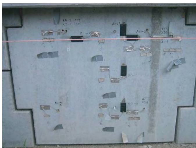
(a) Surface of panel
