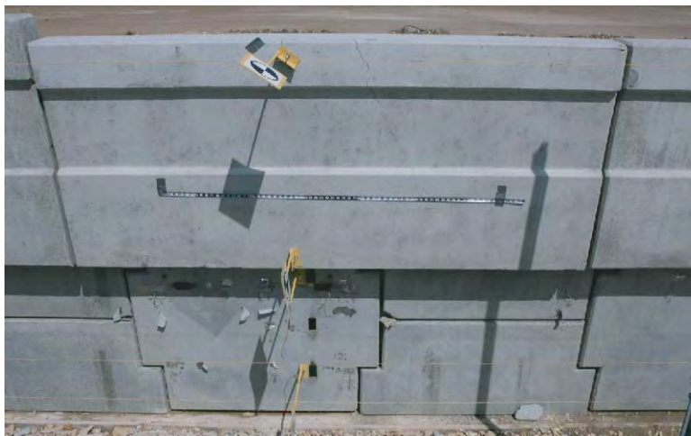
(e) Back view of the barrier
