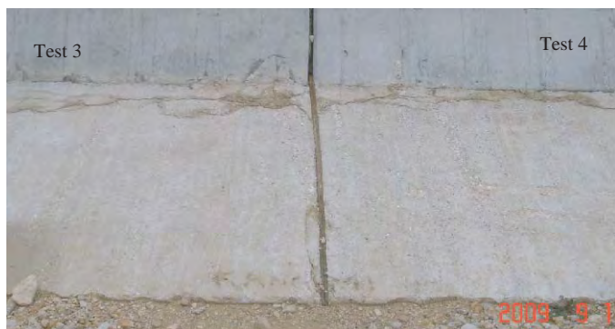
(c) Test 3 and Test 4
