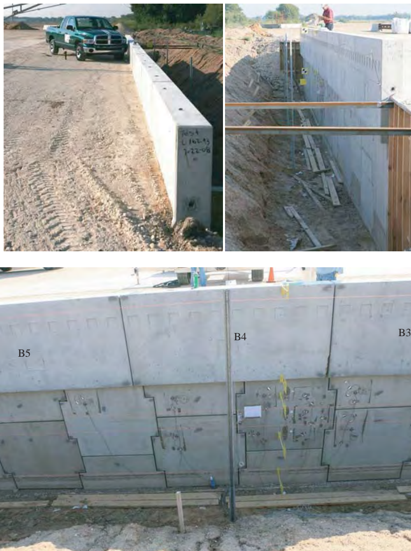
Figure 6.24. Barrier on MSE wall prior to testing.
