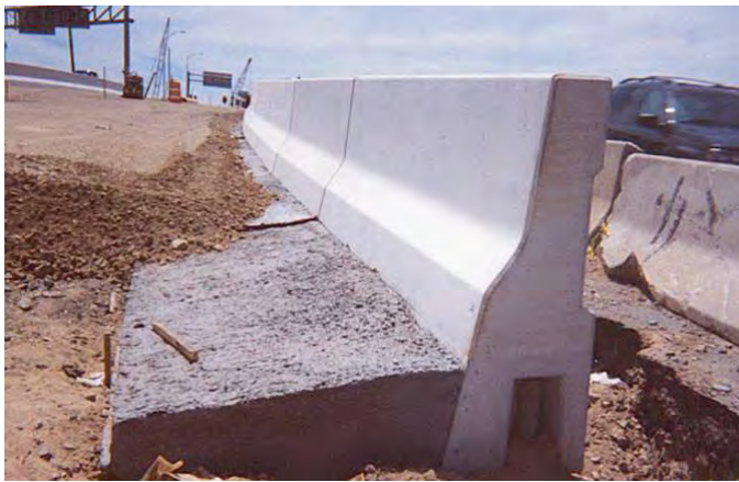
Figure 2.15. Precast barrier and coping with cast-in-place slab.
