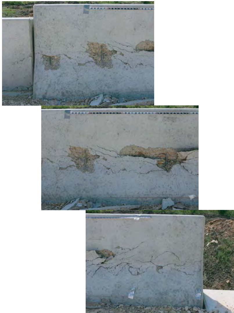
(b) Closeup of front side of the barrier
