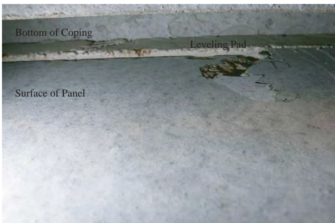
(b) Top of panel inside of recessed coping
