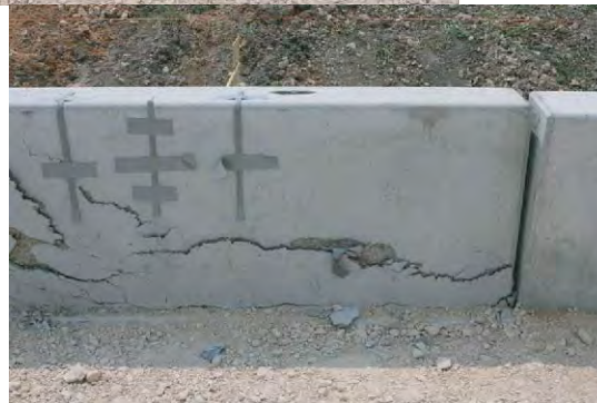
(b) Close-up front side of the barrier
