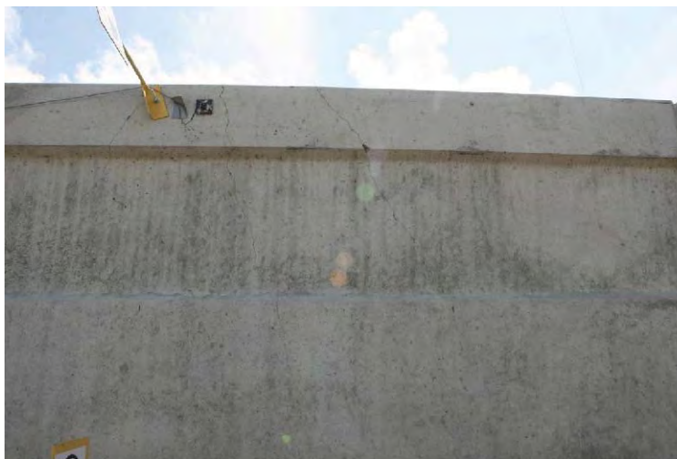
(e) Back view of the barrier
