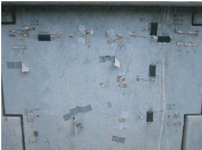
(a) Surface of panel
