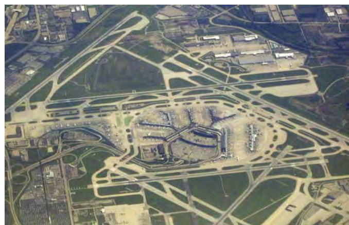
Figure 2.13-1. Aerial view of O’Hare International Airport.
