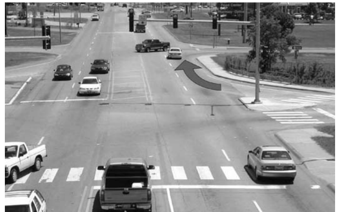
Exhibit 4-4. Driveways too close to exit ramp terminals allow more conflicts to occur.
