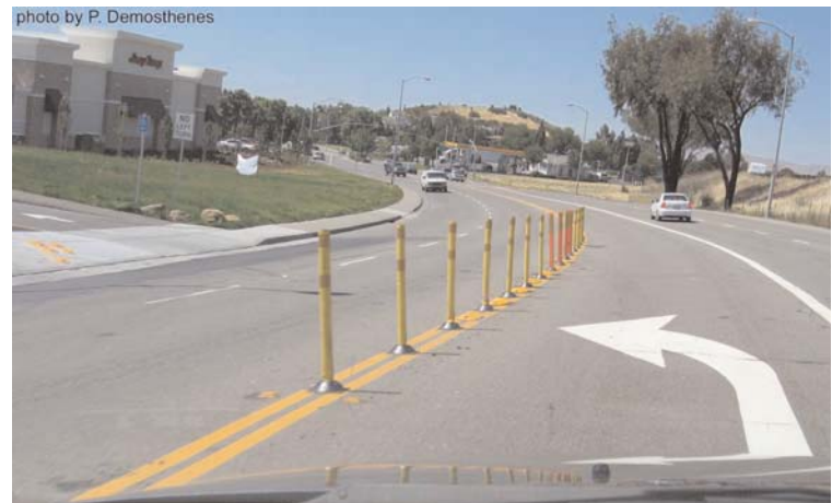
Exhibit 5-83. Example of tubular markers to prohibit a movement.
