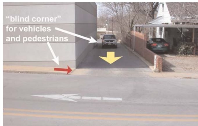
Exhibit 5-11. Driveway with very limited sight distance.
