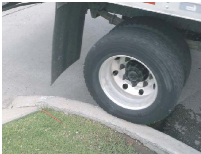
Exhibit 5-15. Effects of inadequate driveway radii.
