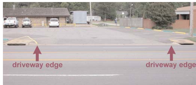
Exhibit 5-48. Drainage inlets too close to the edges of the driveway.
