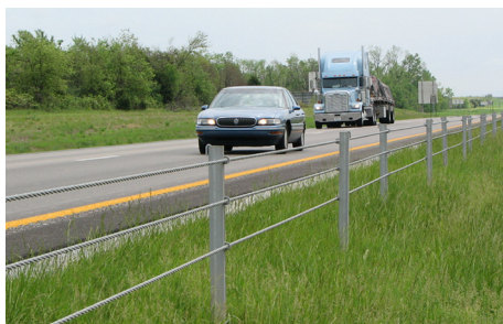
Cable median barrier in Missouri.
