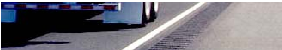
FIGURE 1 Shoulder rumble strips.
