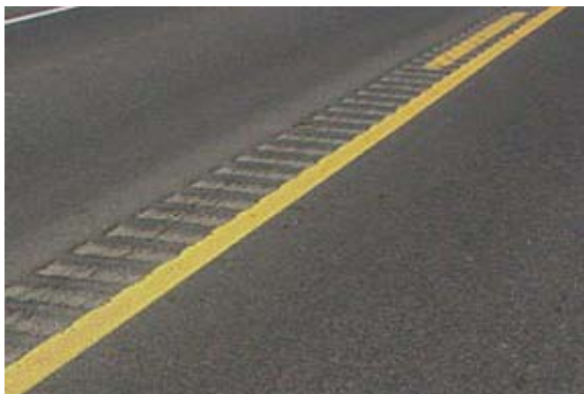
FIGURE 4 Centerline milled rumble strips.
