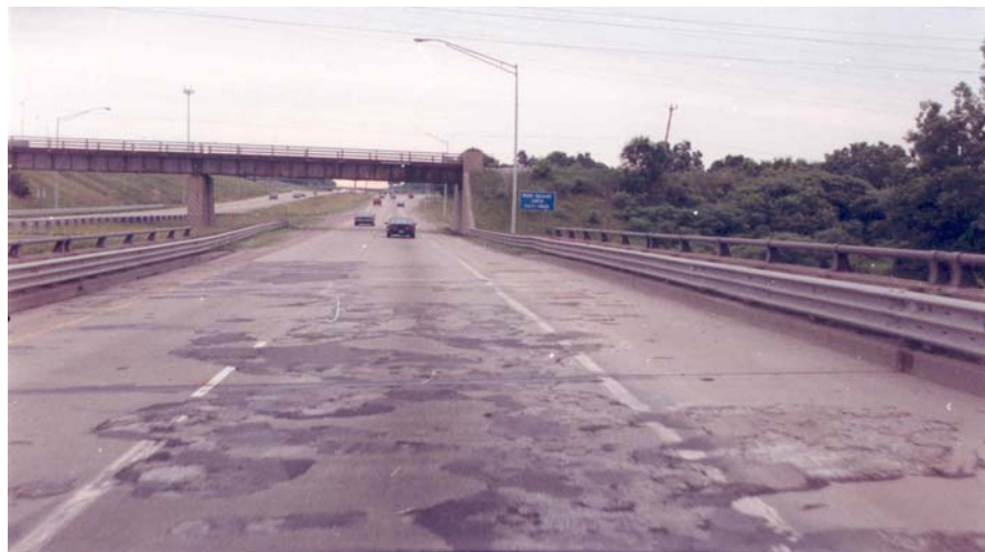
FIGURE 2 Repairs of critical roughness on a concrete bridge deck.
