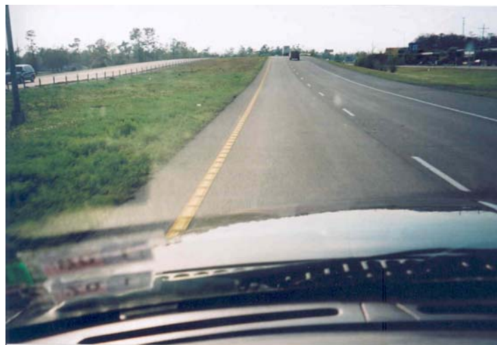
FIGURE 3 Permanent raised pavement markings.
