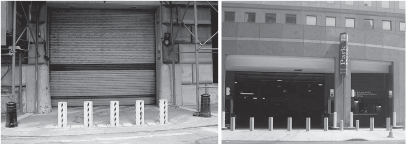
Figure 3-9. Examples of retractable bollards and crash beams.
