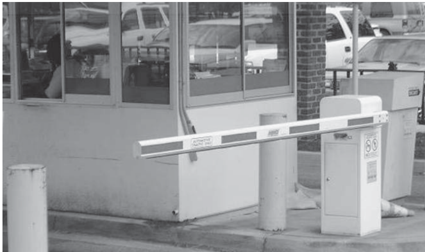
Figure 3-16. Token-based drop arm barrier system.
