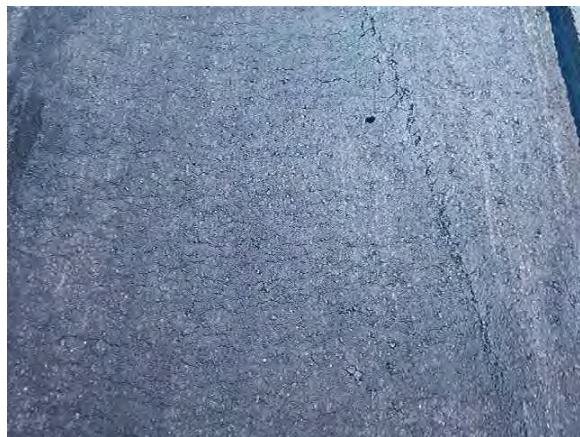
d) Finished surface; checking & mat tears
