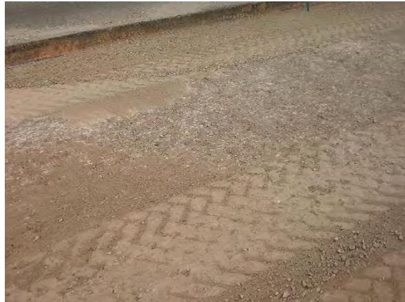
Figure B.67. South Carolina Crushed Granite Base Placed in NCAT Section S-11
