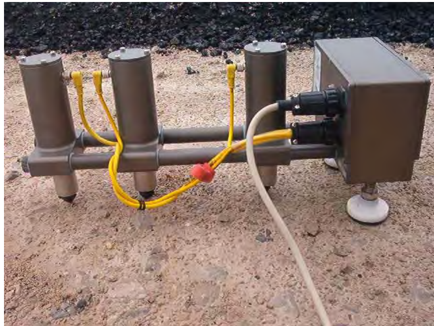
Figure B.83. Seismic Testing of the Crushed Stone Base Layer Along SR-53 New Construction Project in Fremont, Ohio
