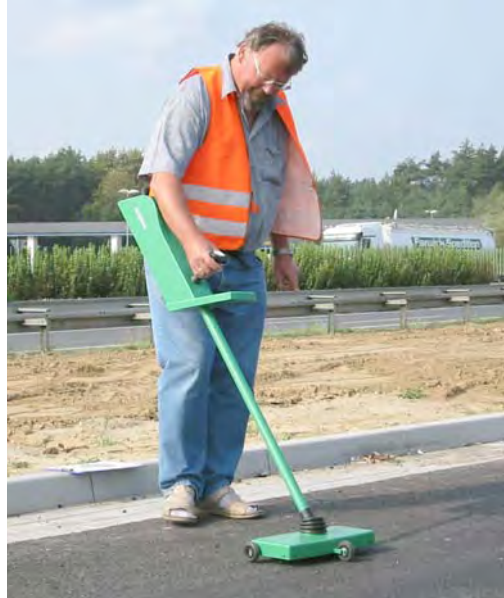
Figure 18. MIT-Scan-T to Measure Flexible Pavement Thickness
