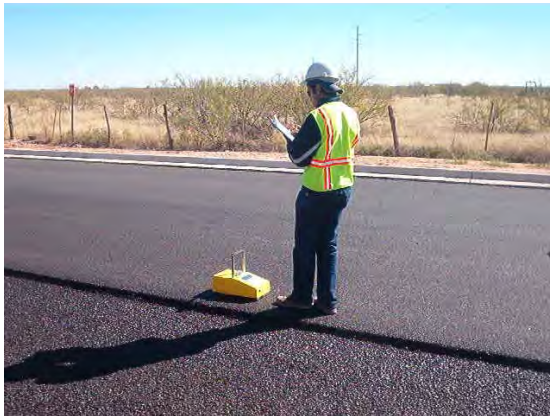
e) Non-nuclear density test
