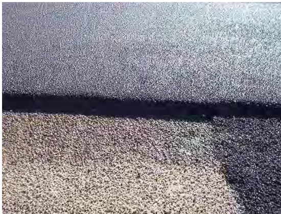
c) Compacted lift
