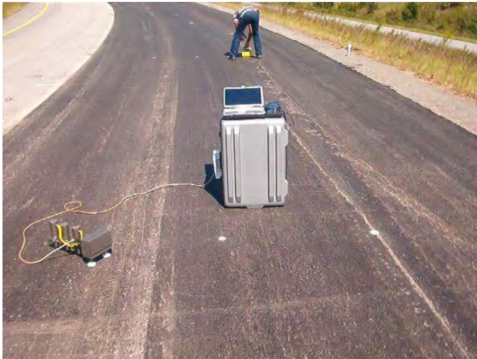
b) NDT testing immediately after paving
