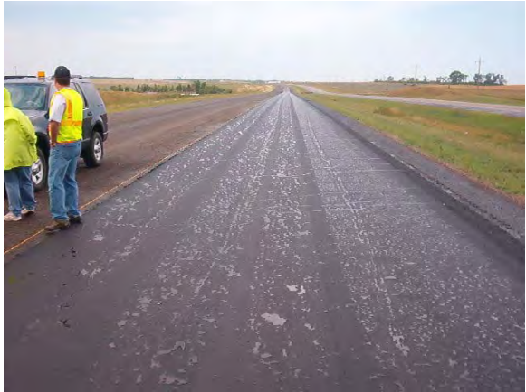
a) Section 1 after rain in 24 hours
