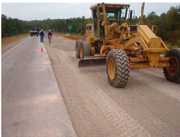
Figure B.67. South Carolina Crushed Granite Base Placed in NCAT Section S-11
