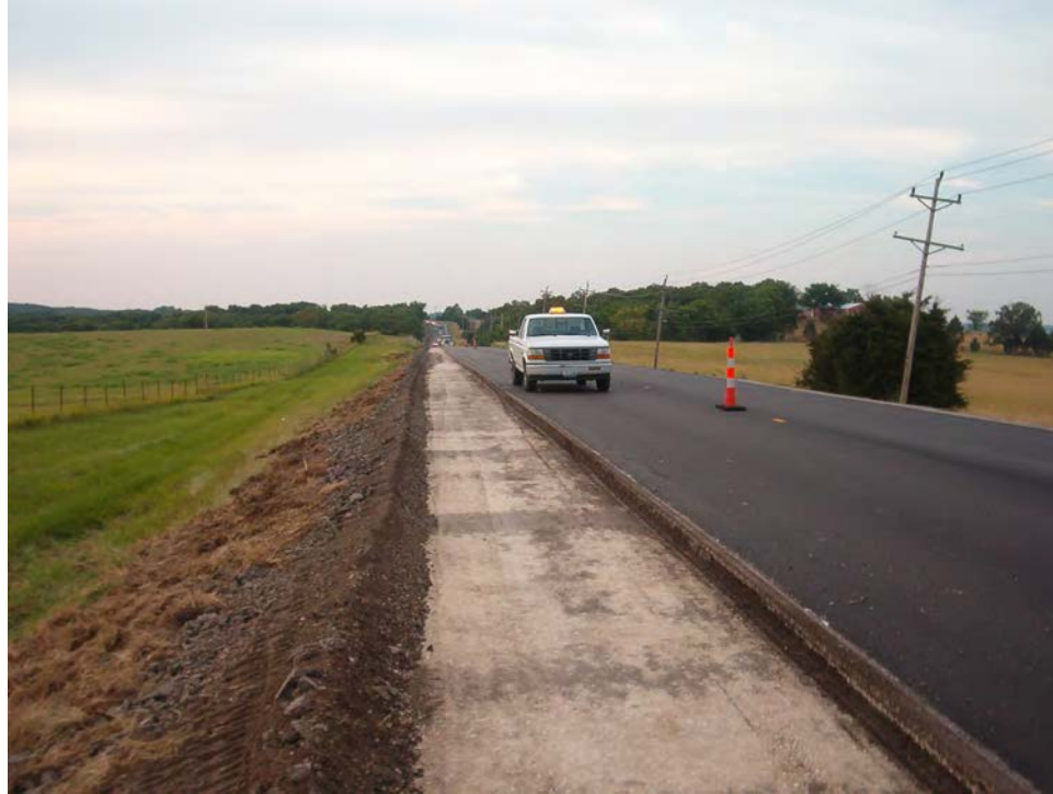
a) Shoulder Condition Before Paving
