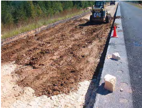
b) Subgrade compaction
