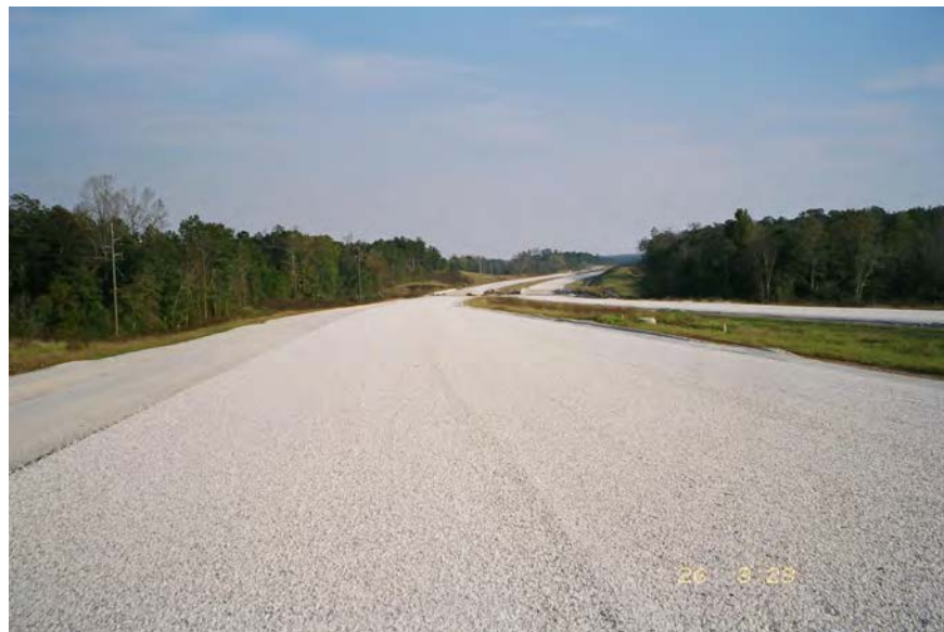
Figure B.10. Crushed Aggregate Base Placed Along US-280 and Used in Part A of the Field Evaluation (refer to Figure B.9); US-280 Viewing East
