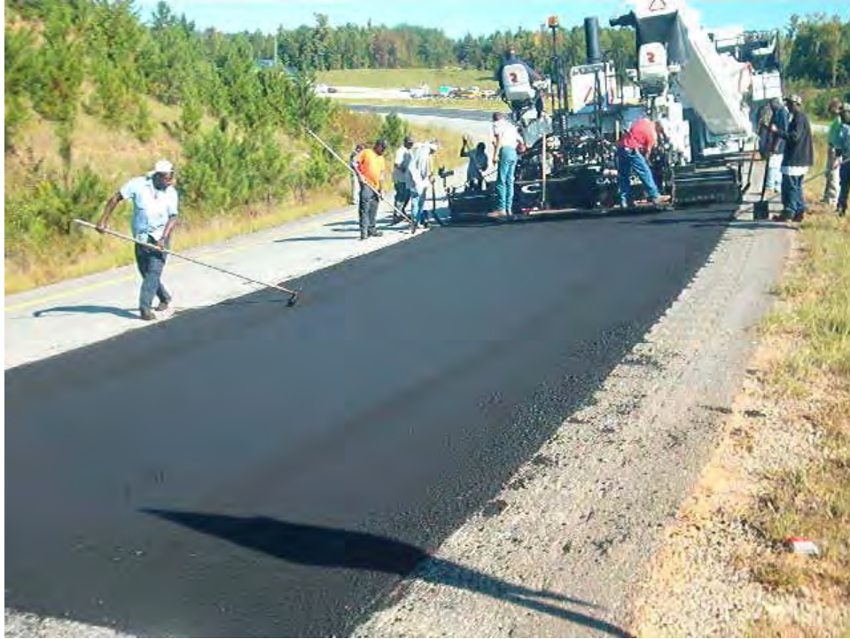
a) Paving of Alabama sections at NCAT test track
