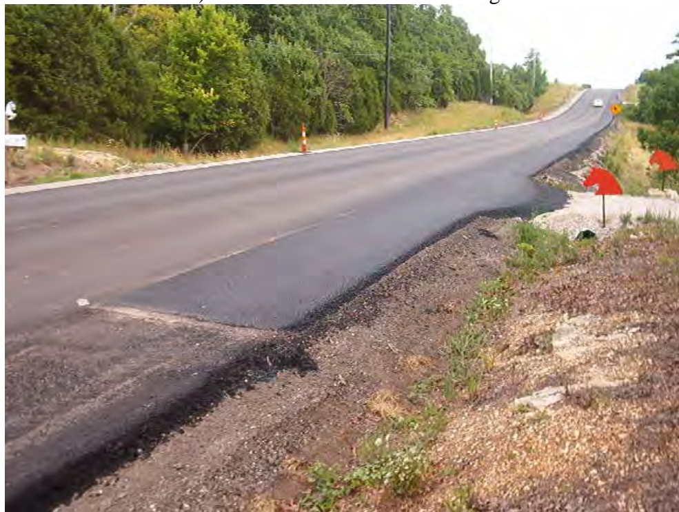
b) Shoulder After Paving
