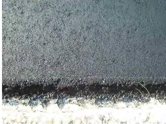
b) Finished surface with first lift
