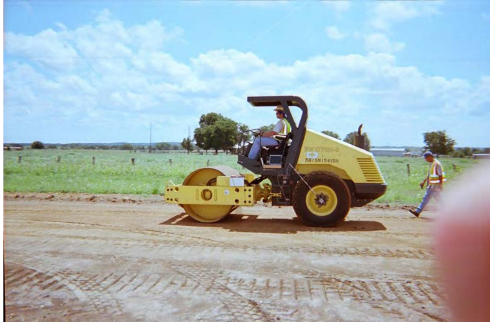
Figure B.24. Roller Used to Compact and Test the Soil Prior to the Use of other NDT Technologies along the Texas SH-21 Widening Project; East of Caldwell, Texas
