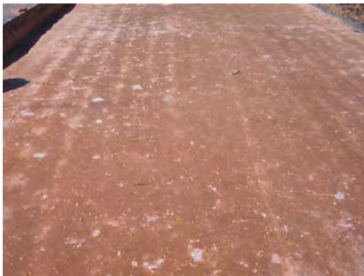
c) Close-up view of compacted base
