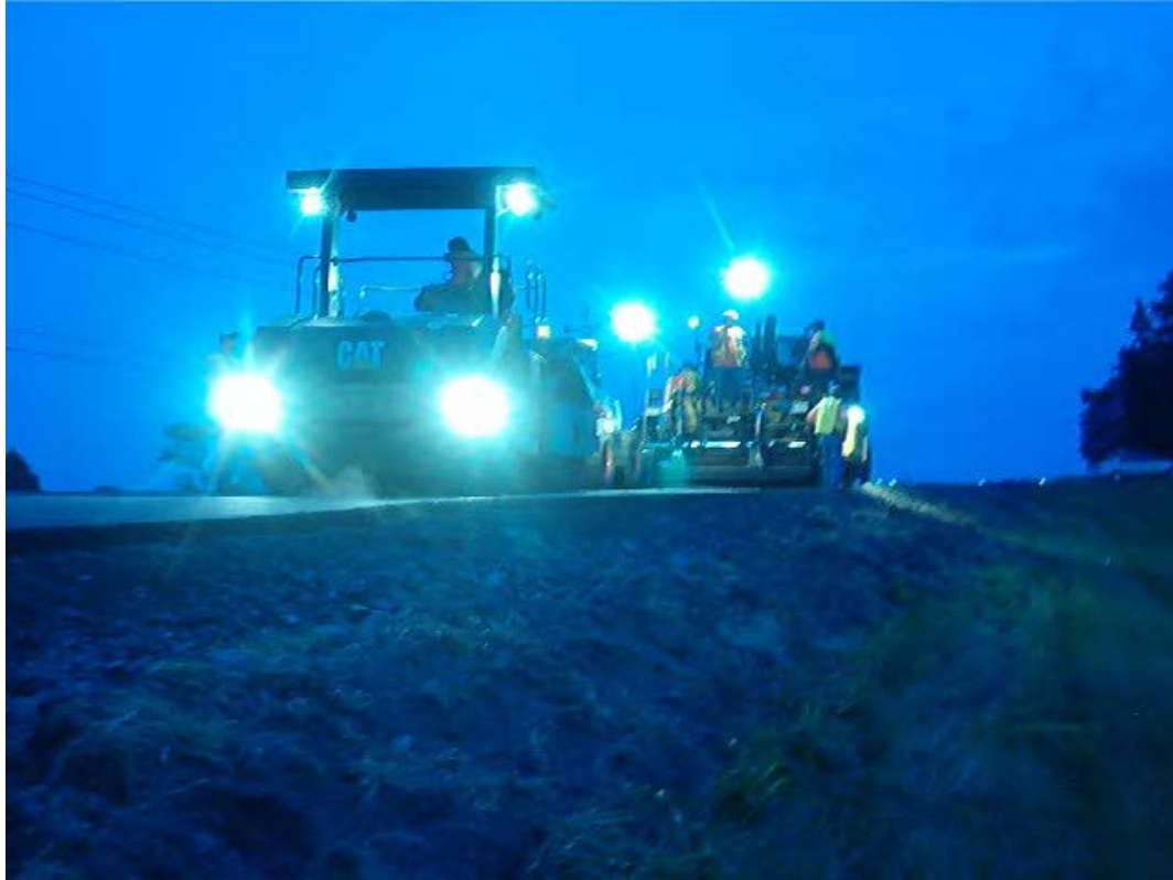
Figure B.27. Nighttime Paving Along US-47, Missouri
