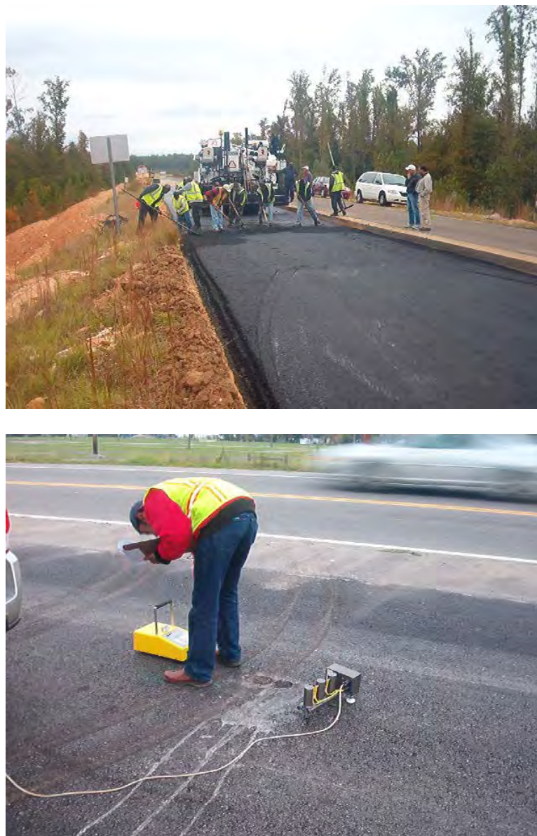
Figure B.85. HMA Paving and NDT Along SR 53 in Ohio
