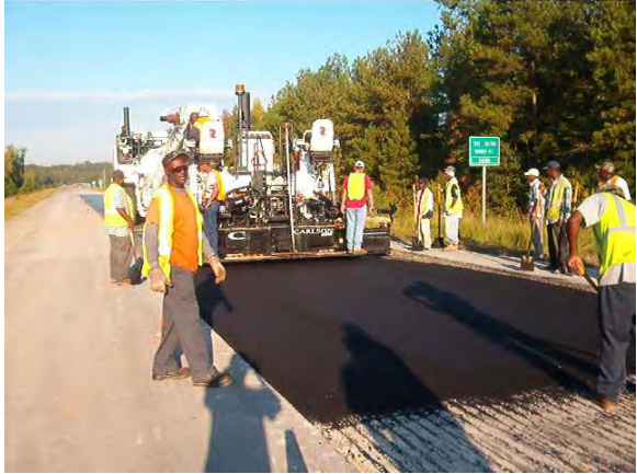
a) Paving first lift
