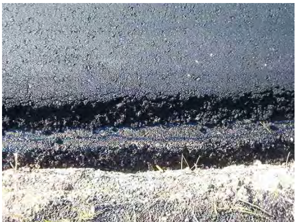
c) Two lift completed
