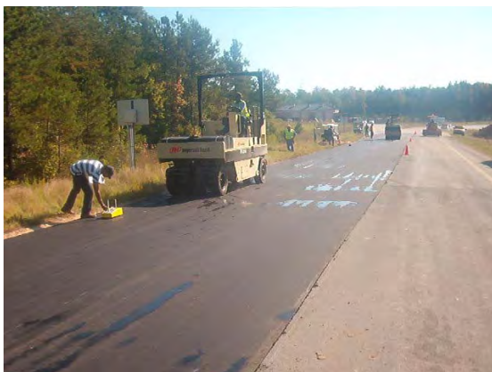
e) NDT testing – Nonnuclear density gage
