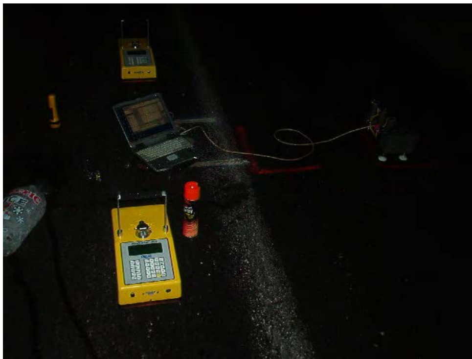
Figure B.30. Multiple Non-nuclear Density Gauge and PSPA Testing on US-47, Missouri
