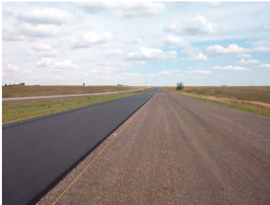
a) HMA paved material for testing
