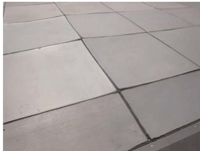
Figure 3-3. MSP Airport: soft tops on EMAS blocks.
