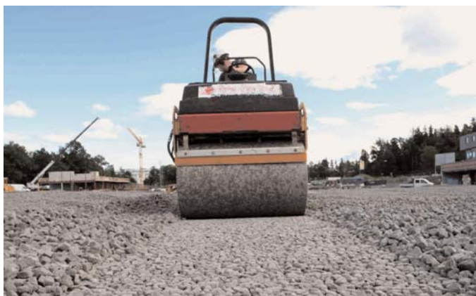
Figure 11-27. Roller compaction of aggregate foam material during typical installation (43).
