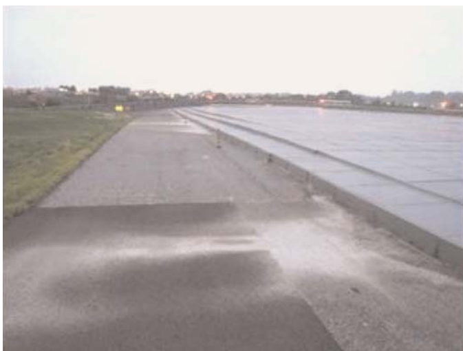
Figure 3-1. LGA arrestor (left) out-washing of material and (right) peeling of joint tape.
