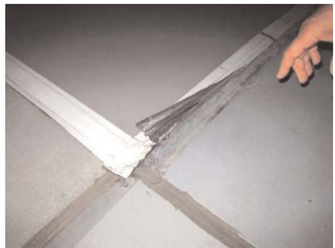
Figure 3-1. LGA arrestor (left) out-washing of material and (right) peeling of joint tape.
