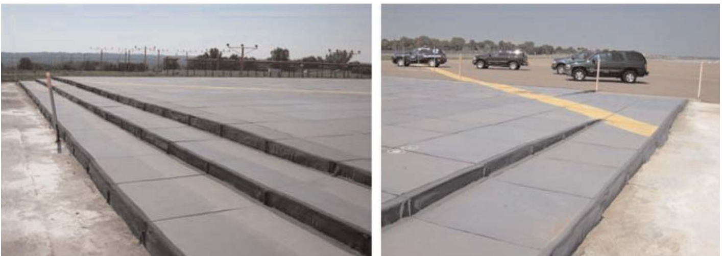
Figure S-1. EMAS arrestor, Minneapolis–St. Paul (MSP) airport.
