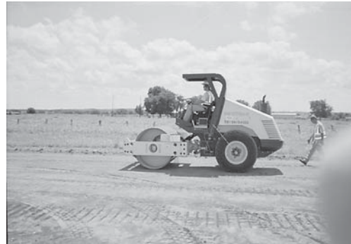
d. Vibratory Roller Instrumented by TTI for Use on Research Projects
