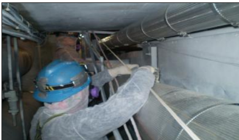
FIGURE 1.5. Workers inside one of the CPP tunnels. SOURCE: AOC
