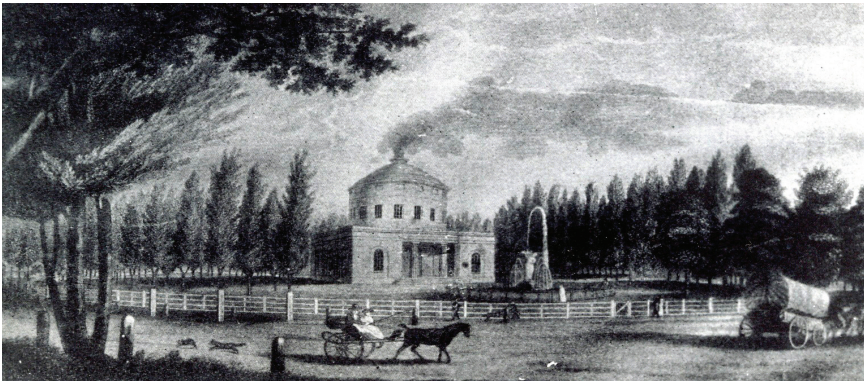
FIGURE 2-1 The Centre Square Pumping Station in Philadelphia in 1801 (early stage of the Fairmount Water Works).
