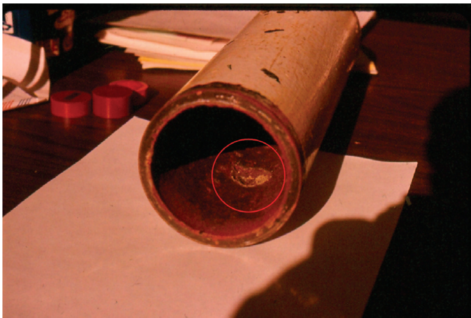
FIGURE 1-4 An internal pit in an oil field water injection pipe. Courtesy of Richard Griffin.
