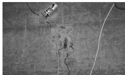
Cracked RCDG bridges were instrumented and monitored.
