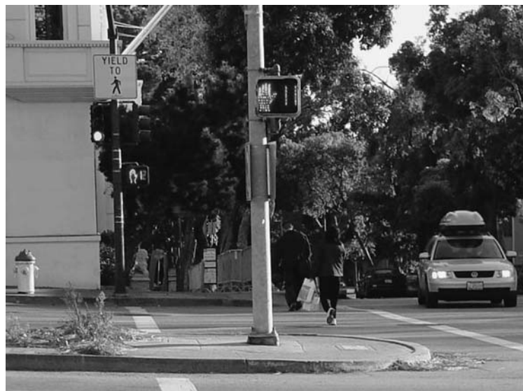
Figure 2-6. Pedestrian countdown signals.
