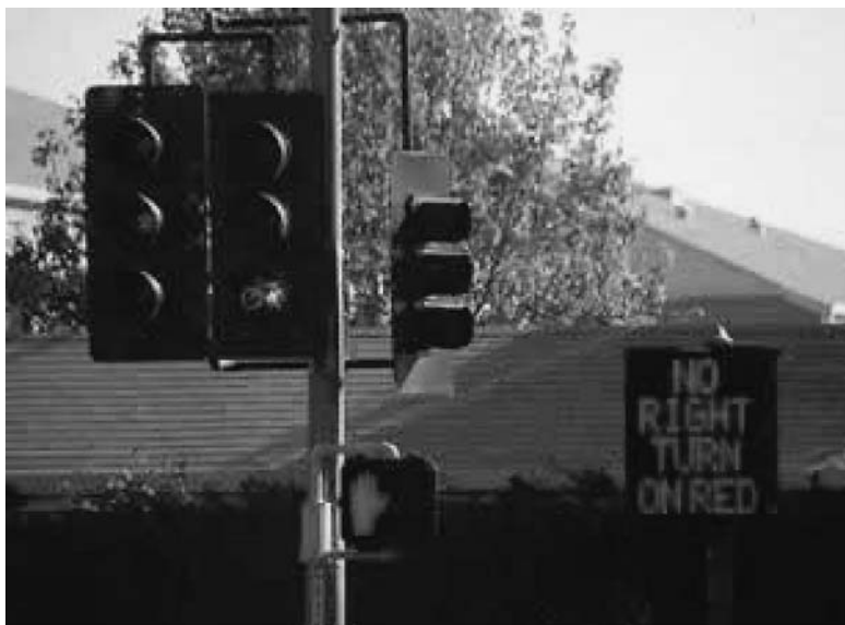
Figure 2-8. Dynamic NO RIGHT TURN ON RED sign.
