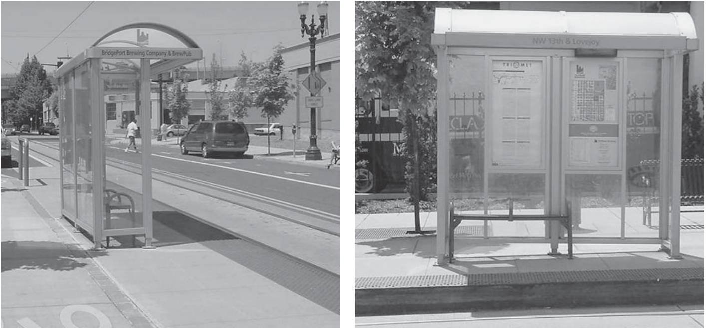
Figure 2-9. Application of tactile strips at a transit stop.
