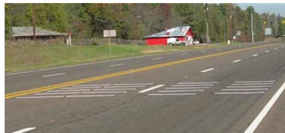
Exhibit 4-15 Northbound on US 271
