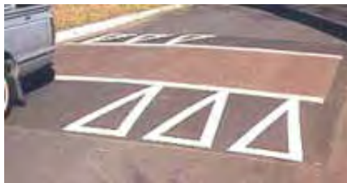
Exhibit 2-25 Speed table combined with striping and colored concrete in Charlotte, NC (Photo: Fehr & Peers)
