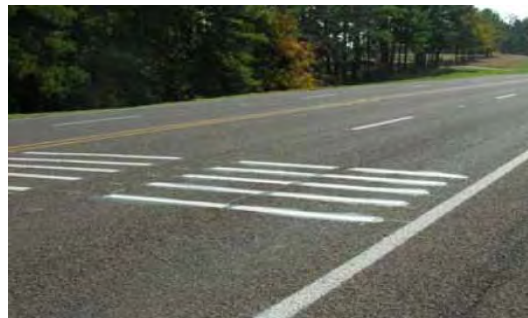
Exhibit 4-13 Southbound on US 271
