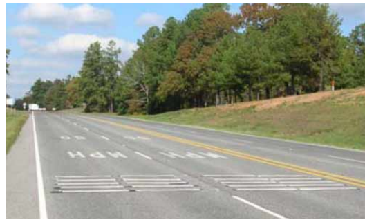
Exhibit 4-12 Southbound on US 271
