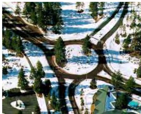
Exhibit 2-15 Single-lane roundabout (Photo: Oregon DOT)
