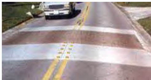
Exhibit 2-24 Speed table combined with textured pavement in Naples, FL (Photo: Fehr & Peers)
