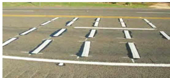
Exhibit 4-17 Northbound on US 271
