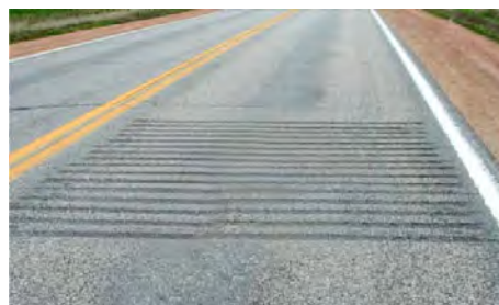
Exhibit 2-10 Transverse Rumble Strips Across the Entire Travel Lane (Photo: Corkle et al.)
