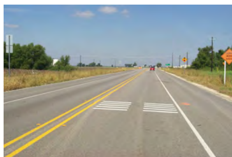
Exhibit 2-8 Transverse Rumble Strips in Wheel Path (TTI)
