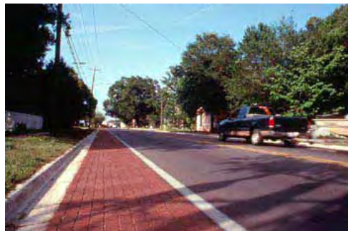
Exhibit 2-28 Example of a shoulder composition application (Photo: Dan Burden)
