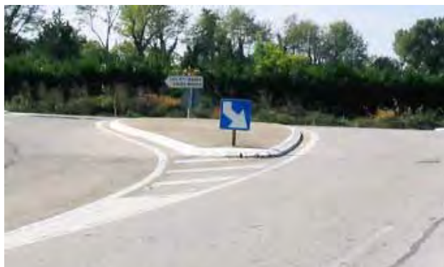
Exhibit 2-20 Splitter Island at a T-intersection in France
