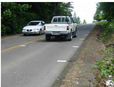
Exhibit 2-7 Peripheral Transverse pavement markings
