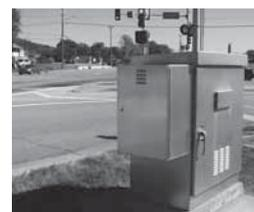
UPS unit and batteries in a piggyback cabinet; the design is suitable for retrofitting a signal cabinet for UPS equipment.
