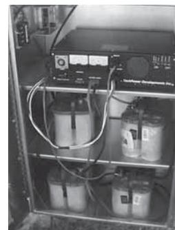
Installation of UPS in a separate, attached cabinet; the UPS unit is on the top shelf, and the batteries are on the middle and bottom shelves.
