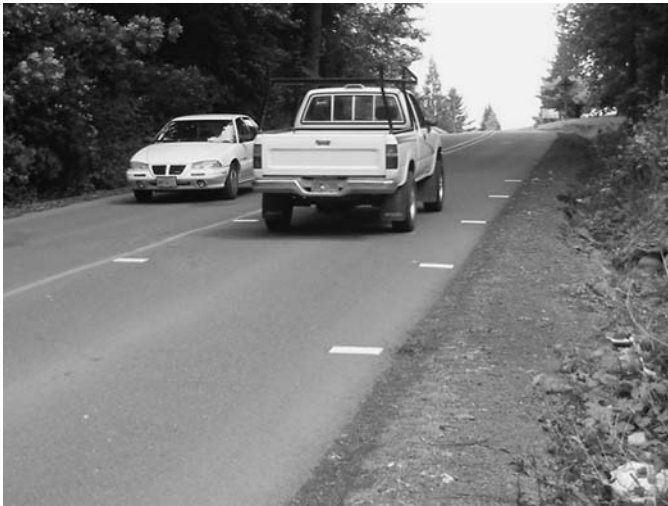
Exhibit B1-7. Eastbound on Whiskey Hill Road near mile post 1.41.
