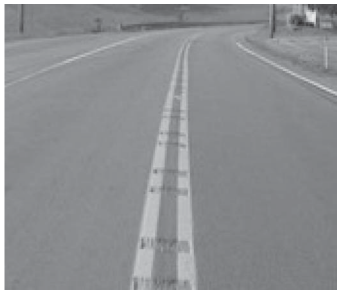
Exhibit 4-9. Centerline rumble strips on the centerline pavement markings.
