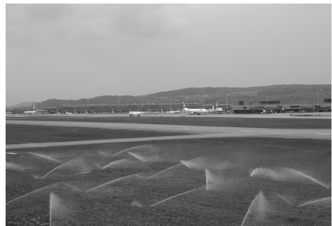
FIGURE 6 Treatment of wastewater from de-icing operations at Zurich Airport.
