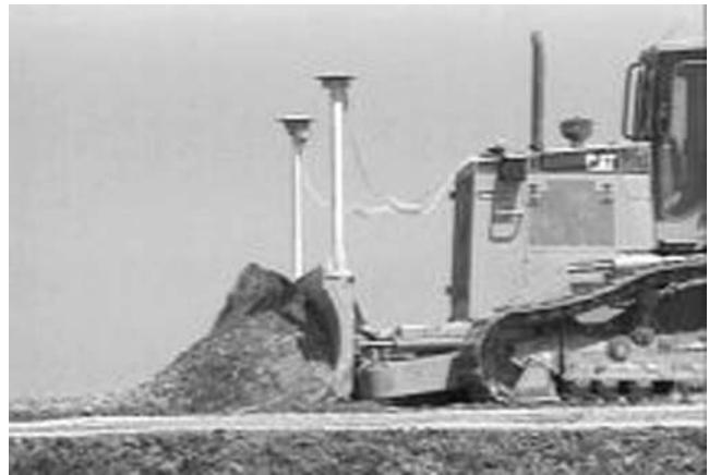
FIGURE 16 Fine grading with GPS-enabled dozer (Courtesy: McAninch Corporation).
