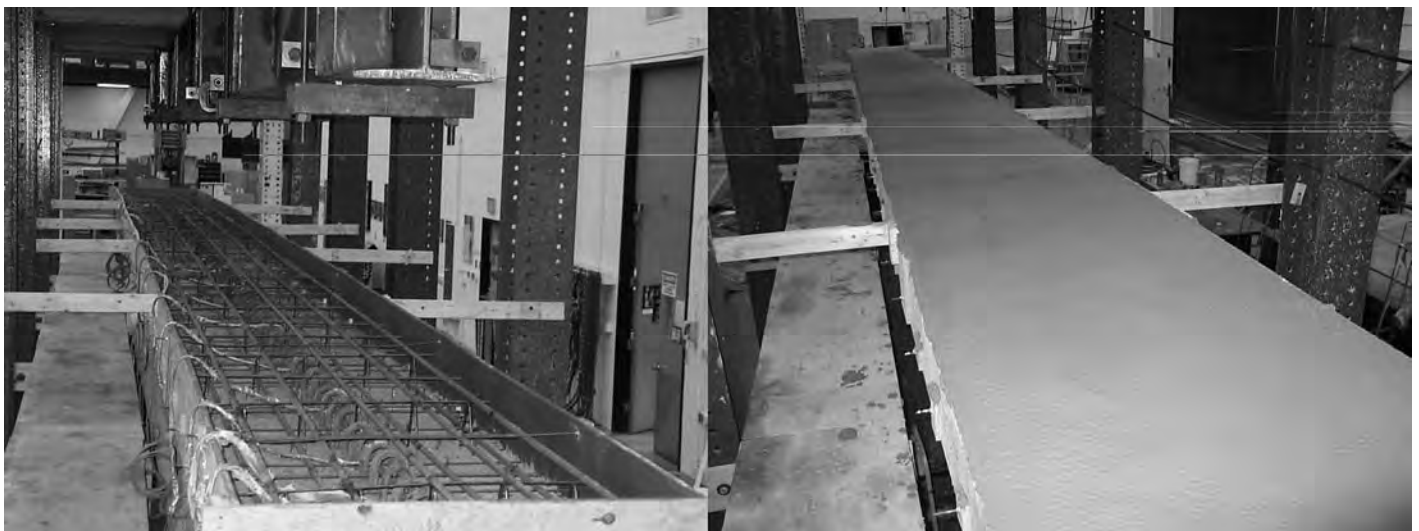
Figure 48. Casting of top deck.
