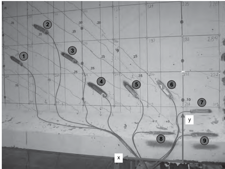
Figure 56. Concrete surface strain gages.
