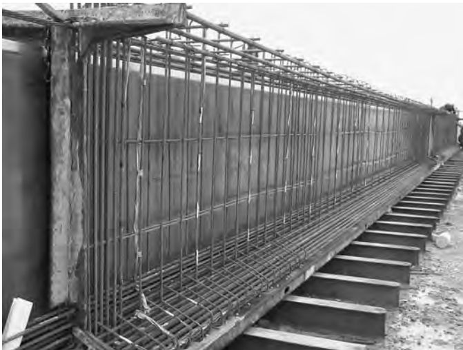
Figure 44. Placement of reinforcement.
