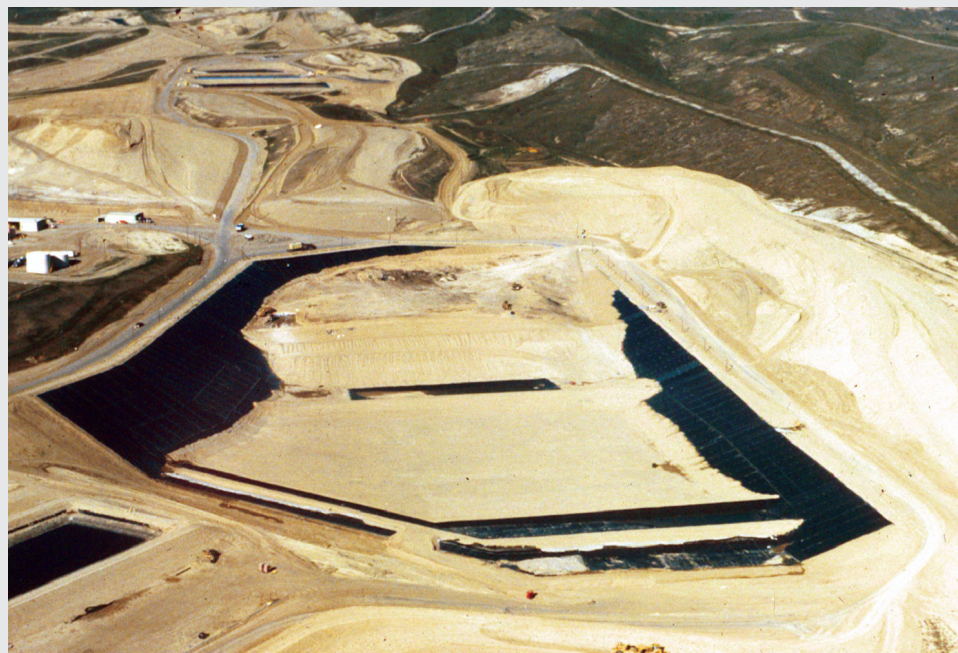
FIGURE 5.11 Kettleman Hills Landfill B-19, Phase 1A, showing waste placed just prior to the stability failure. SOURCE: Golder Associates.
