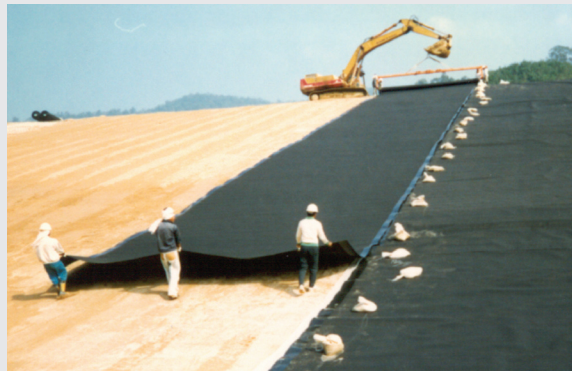
Geomembrane deployment on a slope. SOURCE: GSE Lining Technology, Inc.
