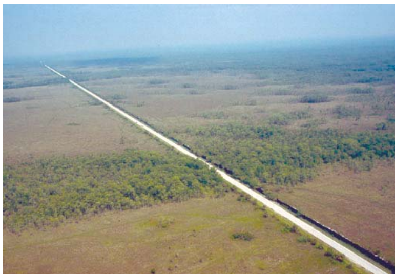
FIGURE 2-6 Built in the 1920s, the two-lane Tamiami Trail (and the adjacent levee L-29) interrupts the natural north-south flow of water through Big Cypress National Preserve and Everglades National Park.
