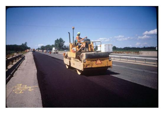
FIGURE 19 Compaction of the longitudinal joint from the hot side.
