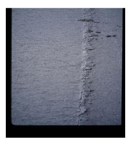
FIGURE 3 Checking of a tender mix.
