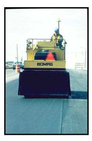
FIGURE 8 Use of rubber tire roller for compacting joint.
