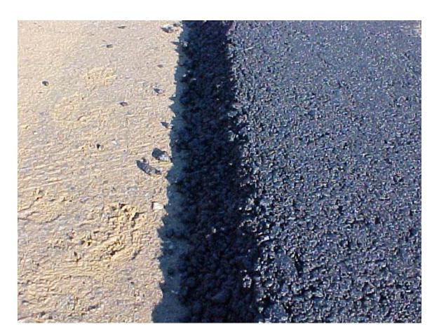
FIGURE 20 Longitudinal wedge joint.
