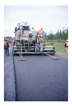
FIGURE 10 Paver placing unsupported edge of pavement.
