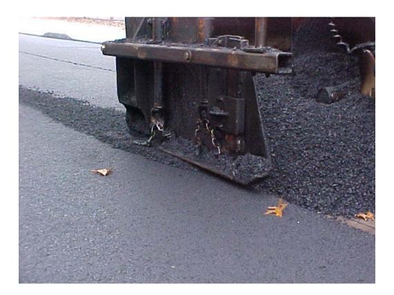
FIGURE 13 Improper placement of the edger plate results in too much overlap.
