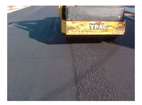
FIGURE 15 Improper raking of the longitudinal joint.
