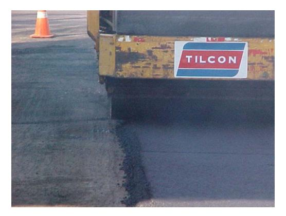
FIGURE 3 The shape of the wedge inhibits proper compaction.
