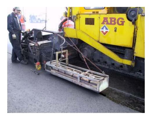
FIGURE 3 Use of joint heaters at longitudinal joints.
