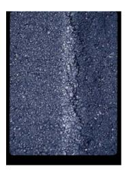
FIGURE 2 Humping up of the mix at the edge of a steel wheel roller drum.
