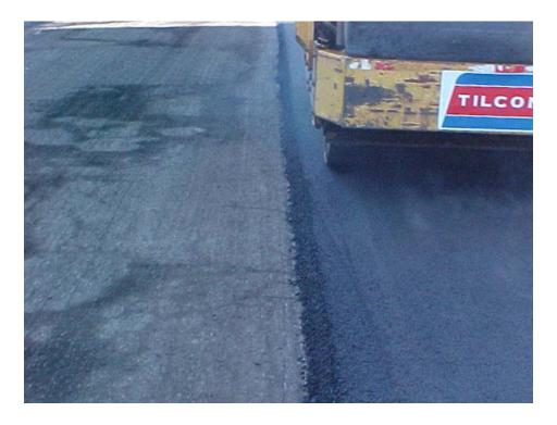
FIGURE 5 Edge of the roller drum inside the unsupported edge of pavement.
