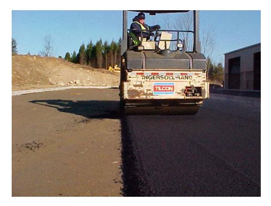
FIGURE 7 Edge of the roller drum directly on the unsupported edge of pavement.
