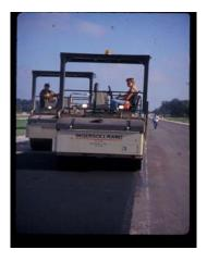
FIGURE 4 Two DDV rollers in echelon behind the paver.
