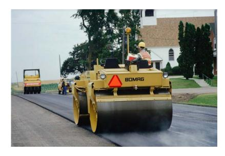
FIGURE 9 Edge of the roller drum extended over the unsupported edge of pavement.
