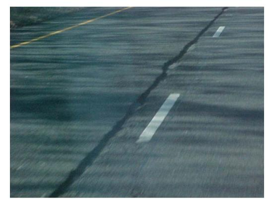
FIGURE 2 Severe erosion of mix at a longitudinal joint.
