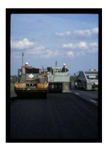
FIGURE 1 Pneumatic tire breakdown roller and DDV finish roller.
