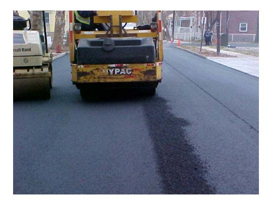
FIGURE 17 Compaction of the longitudinal joint from the cold side.
