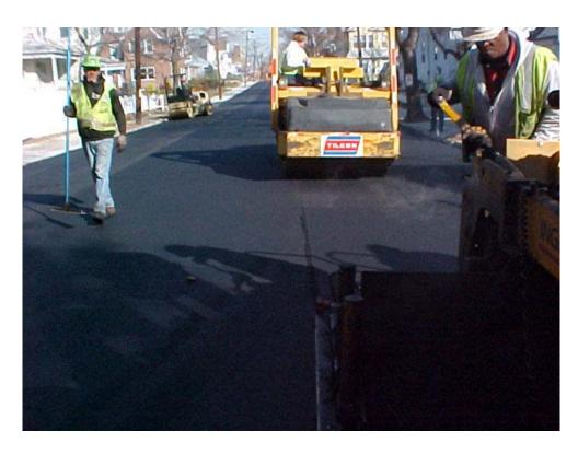
FIGURE 16 Proper raking at the joint (note location of rake).
