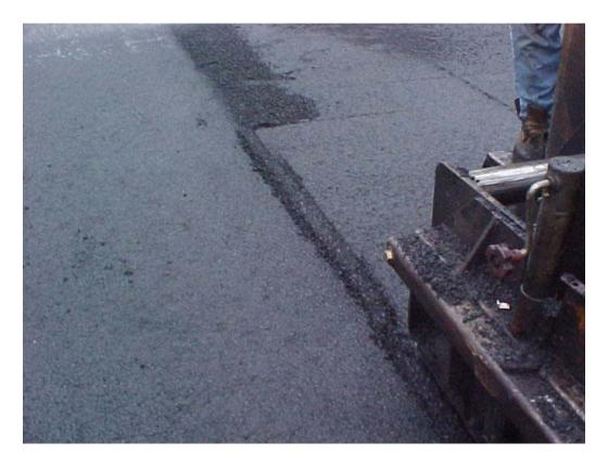
FIGURE 12 Excessive amount of overlap mix from Lane 2 over Lane 1, which creates the need for improper raking of the joint.
