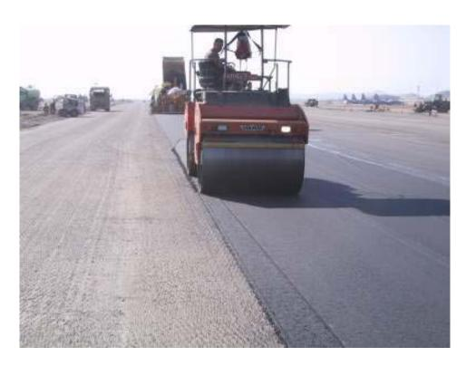
FIGURE 2 Breaking over of material at edge when rolling.
