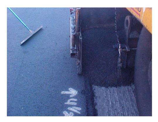
FIGURE 14 Proper amount of overlap of mix from Lane 2 over Lane 1.
