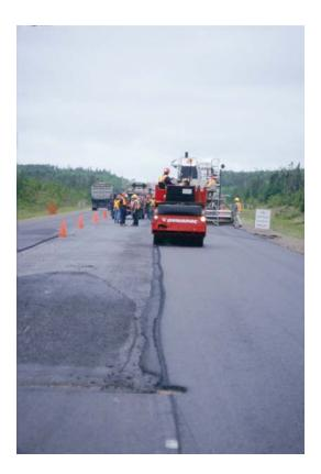
FIGURE 11 Transverse movement of the mix at the unsupported edge of pavement.
