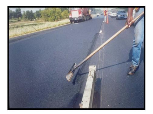
FIGURE 6 Luting of longitudinal joint.
