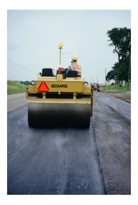
FIGURE 4 Edge of the roller drum inside the unsupported edge of pavement.
