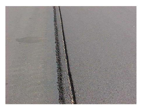
FIGURE 5 Cutting back of free edge.
