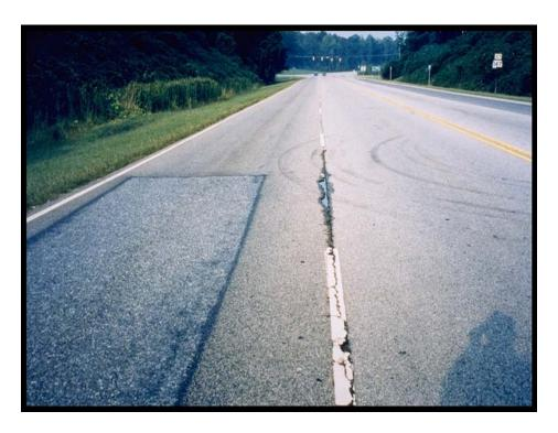
FIGURE 1 Opening of longitudinal joint.
