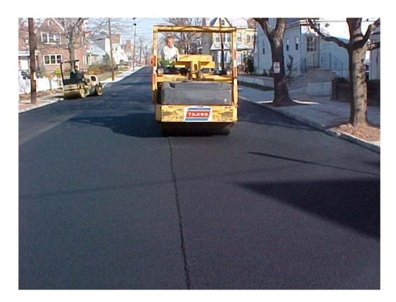
FIGURE 18 Compaction of the longitudinal joint from the hot side.
