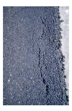
FIGURE 6 Crack formed from rolling inside the edge of pavement.
