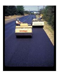
FIGURE 5 Two DDV rollers in echelon behind the paver.
