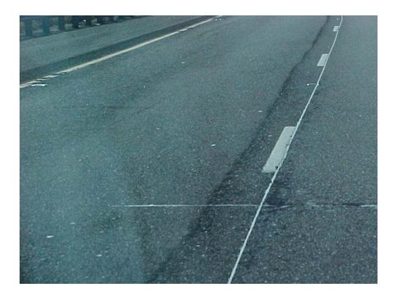
FIGURE 1 Raveling at a longitudinal joint.
