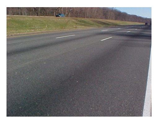
FIGURE 22 New Jersey Route 80, paved in 1992, with joints still in good condition.
