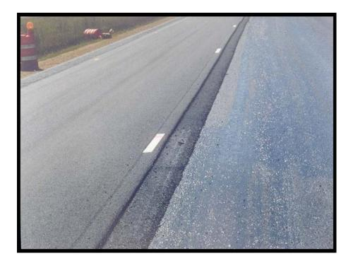
FIGURE 9 Notched wedge joint.
