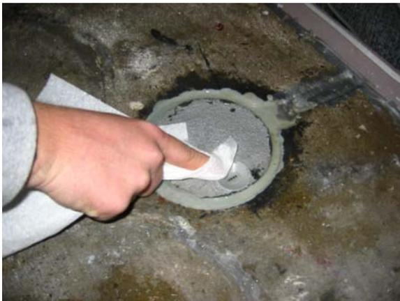
*Figure 3-1. Cleaning Pavement Sensor Depression with Paper Towel.*
