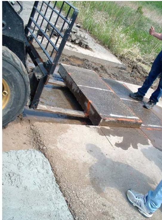
**Figure 7. Removal of the Asphalt Test Section at Mn/DOT's Mn/ROAD Facility**
