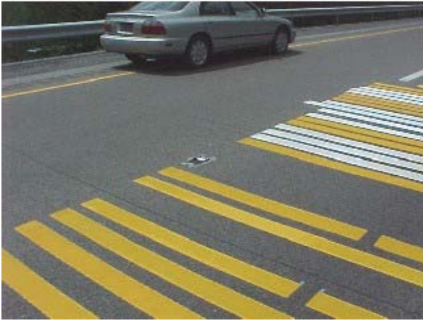
Figure 5. ASTM D713 field test for pavement marking material (24)
