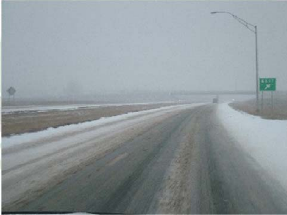
FIGURE 8 Photo of transition.
