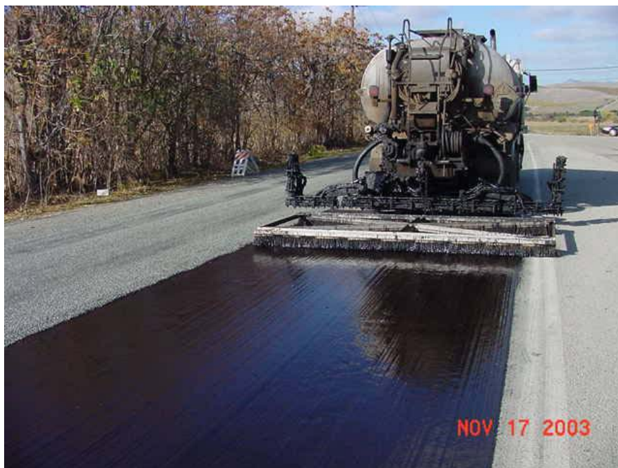
FIGURE 6 Scrub seal application.
