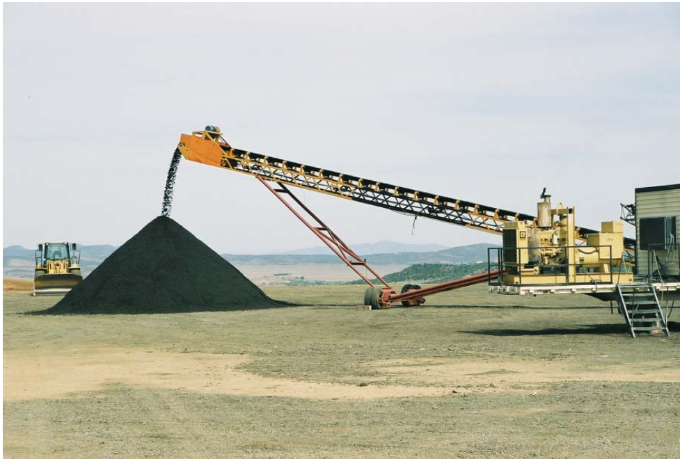
FIGURE 3 Central plant-mixed (pugmill) emulsion mix.
