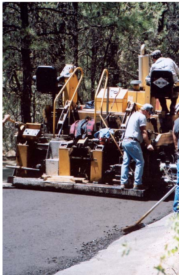
FIGURE 4 Dense-graded emulsion mix, paver laid.
