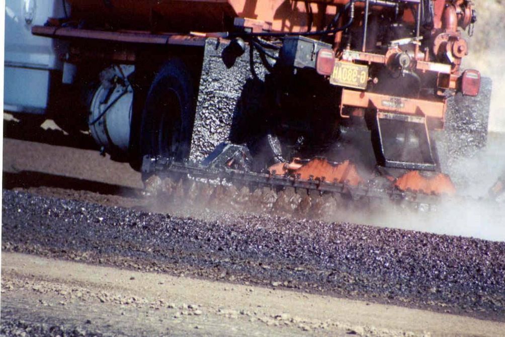
FIGURE 2 Emulsion mix mixing table.
