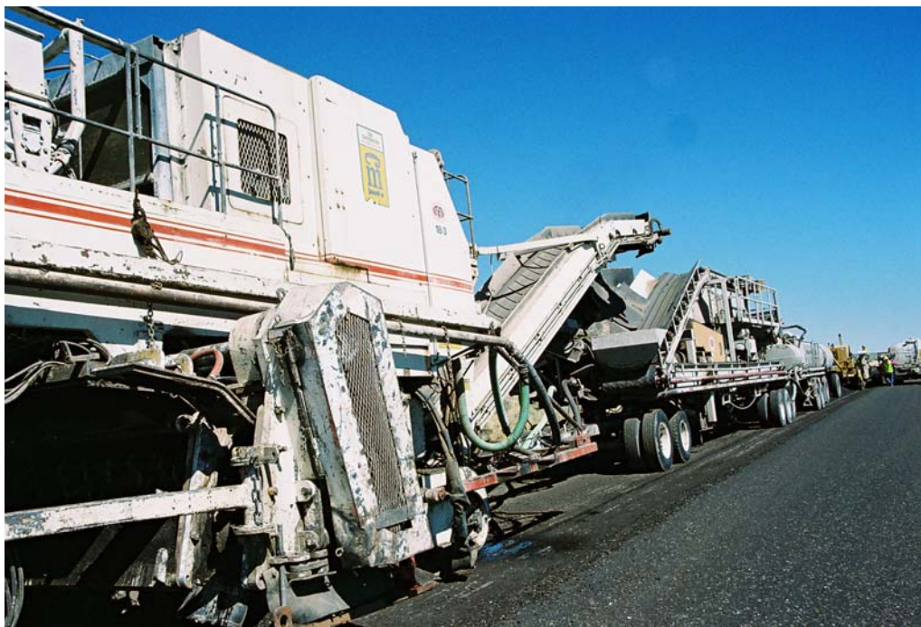
FIGURE 24 Cold in-place recycling train.
