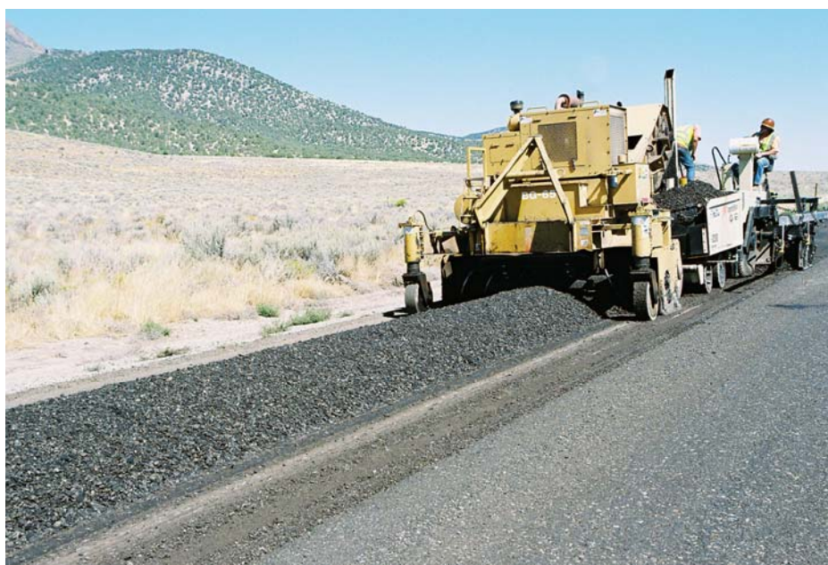
FIGURE 5 Windrow laydown, paver-laid emulsion mix.
