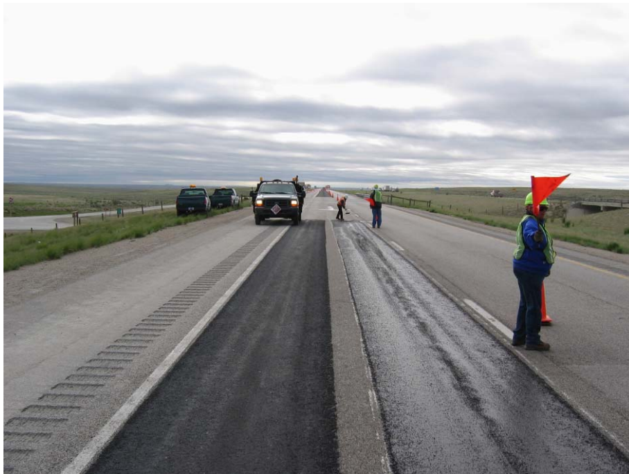
FIGURE 16 Rut-filling application of microsurfacing.
