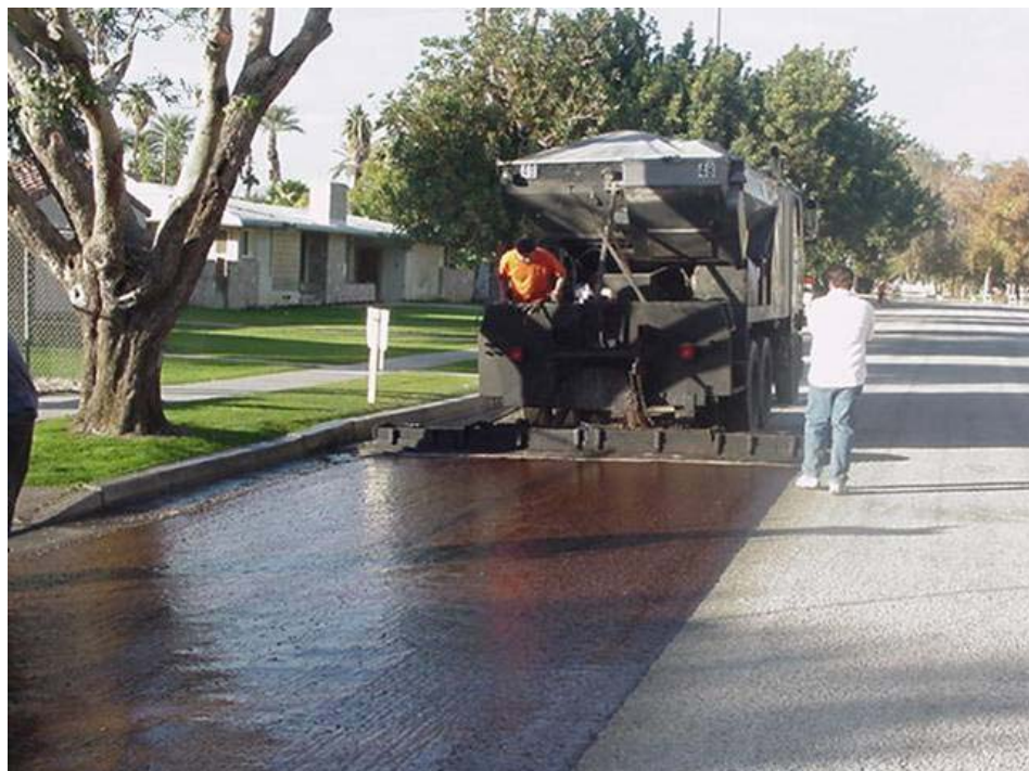
FIGURE 17 Type II slurry being applied on a cape scrub seal.
