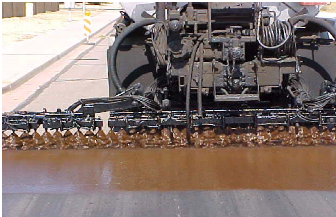
FIGURE 1 Tack coat application.
