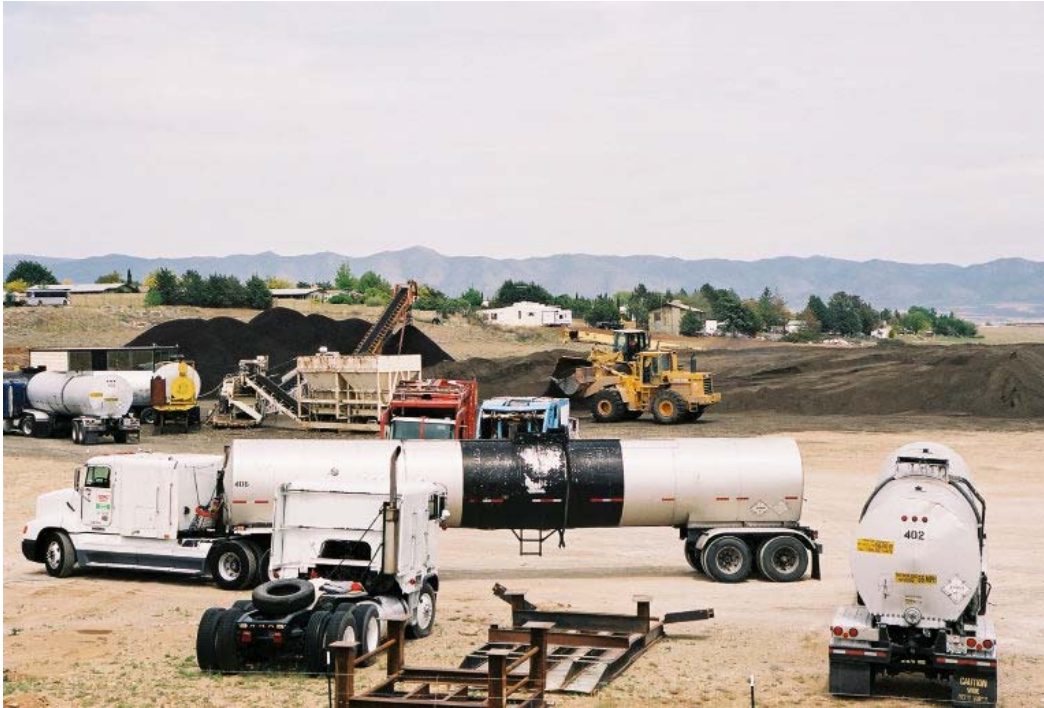
FIGURE 22 On-site mixing of RAP emulsion mix.
