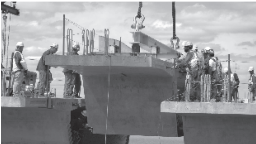
Workers position the final segment of the new Four Bears Bridge.
