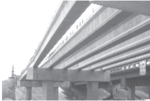
HPC girders of the Jonesboro Road Bridge during construction.
