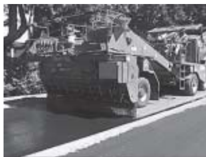
Applying chip seal to preserve a highway surface.
