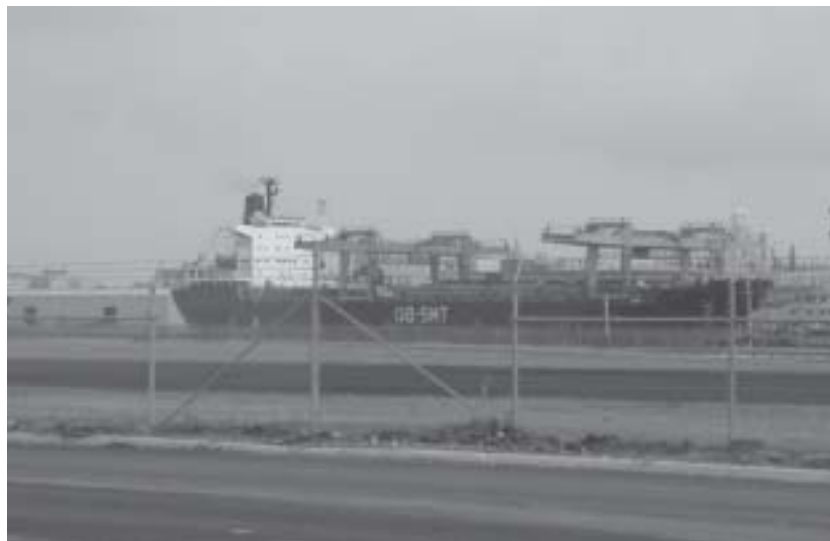
Containership in the Port of San Juan, Puerto Rico.
