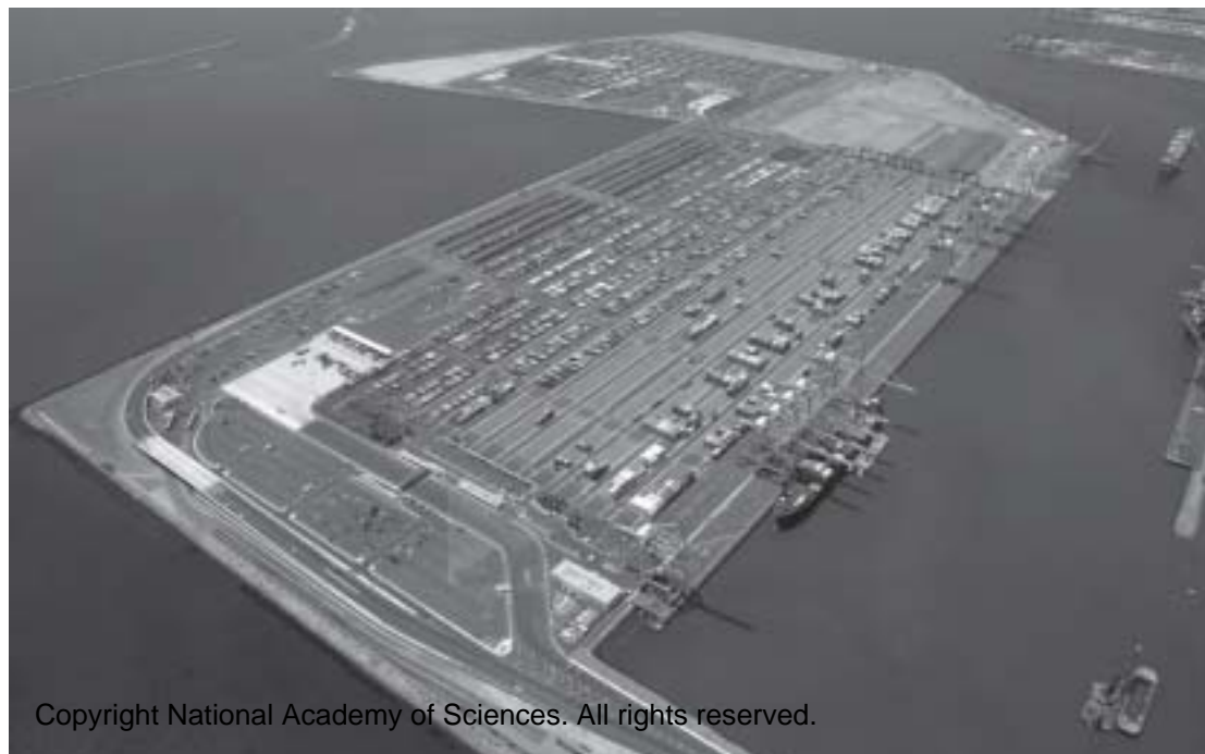
PHOTO: PORT OF LOS ANGELES
