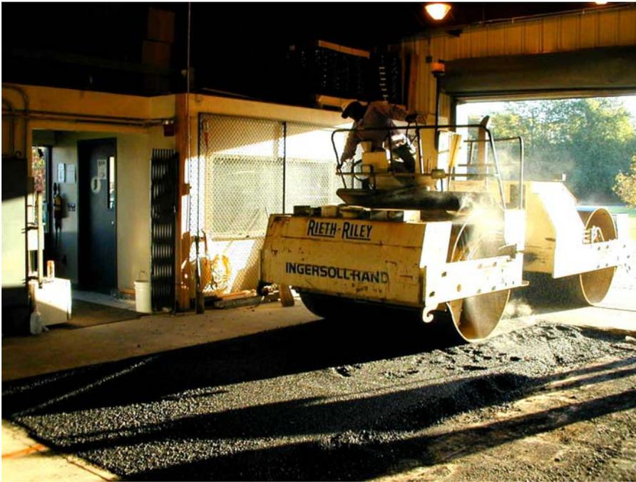
Figure D.5 Mixture compaction
