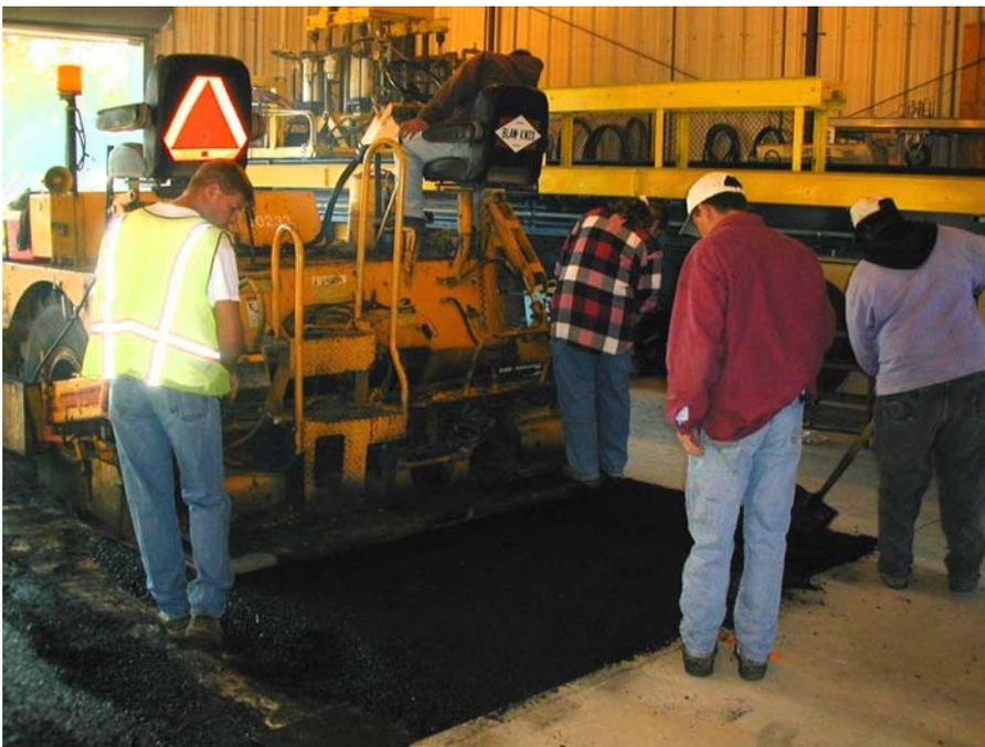
Figure D.4 Test section paving
