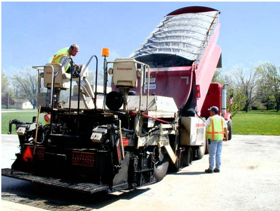
Figure D.2 Loading the paver
