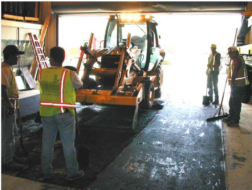
Figure D.6 Center section is removed
