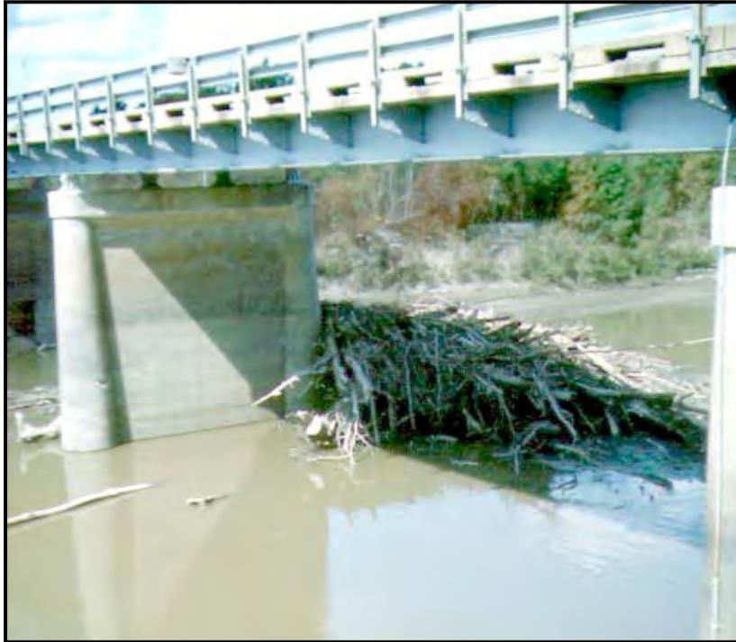
*Figure 2. – Looking upstream at the remnants of the debris raft formed in front of the middle pier (#2) of the S.R. 129 bridge over the Chariton River during the May 24, 1995 flood.*
