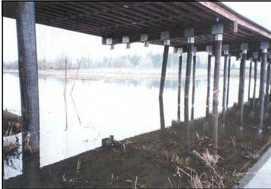
*Figure 9. Looking east at failed pier #9 following the February 1996 flood.*
