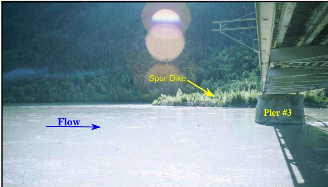
*Figure 10. Looking along upstream face of the old Old Glen Highway bridge over the Knik River at the left bank and spur dike.*
