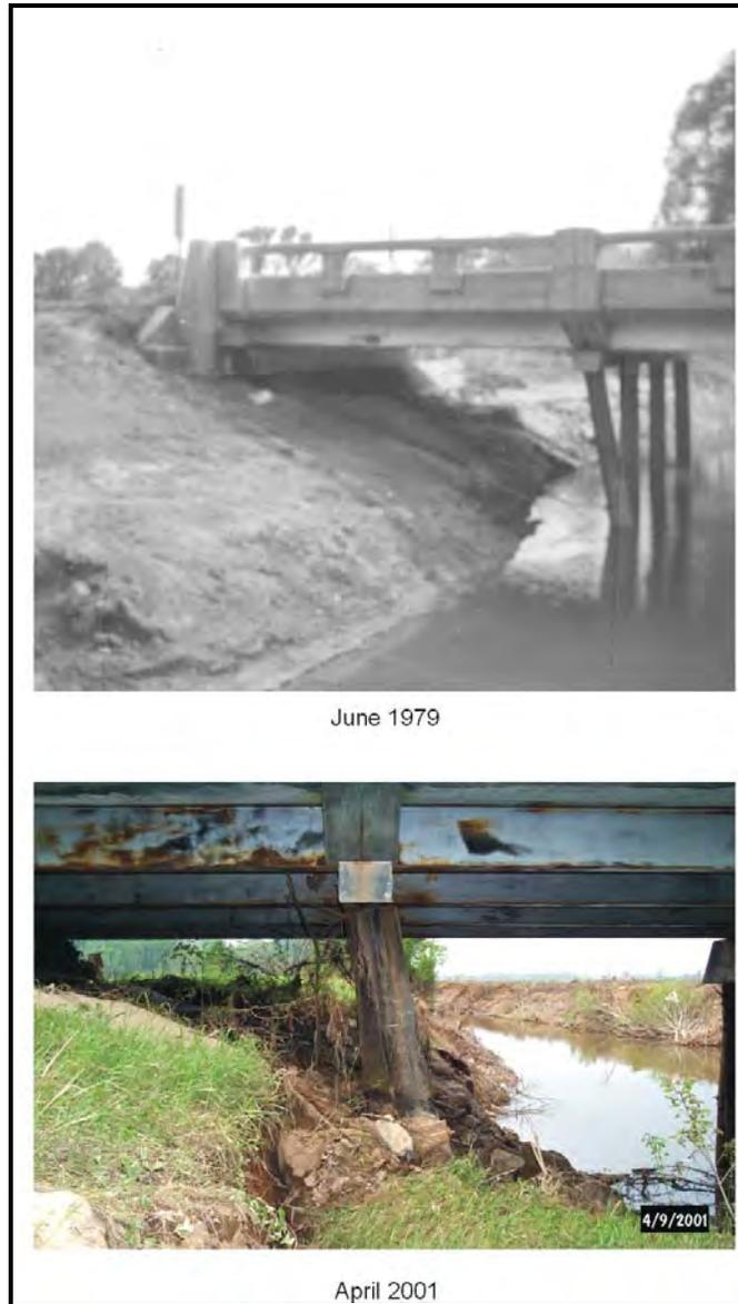
**Figure 7.** Looking downstream through the S.R. 35 bridge opening at left abutment and pile bent no. 2 following the 1979 and 2001 floods on Conehoma Creek.
