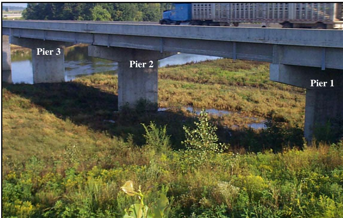
*Figure 12. Looking upstream at left overbank and areas of clear-water scour from downstream US 218 bridge over Cedar River during low flow, 8/10/99.*
