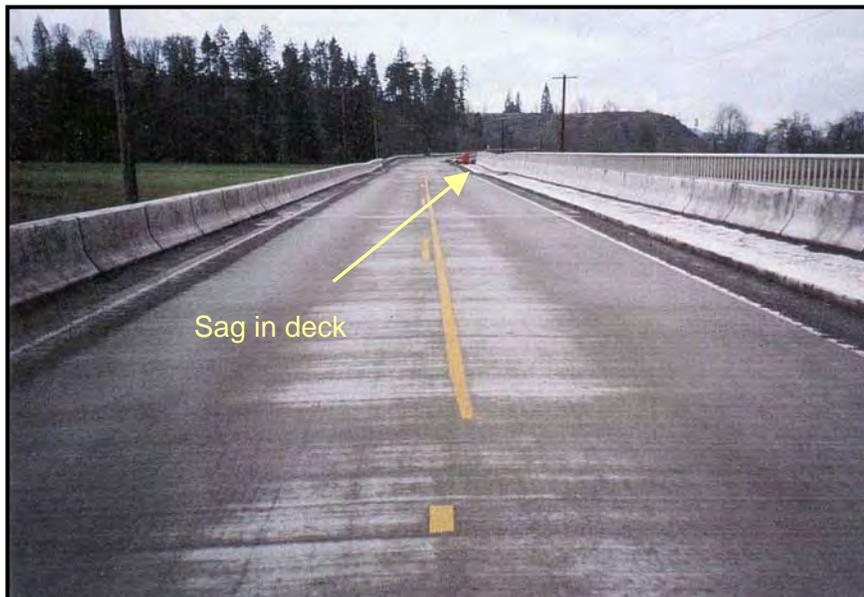
*Figure 10. Looking west toward sag in bridge deck due to failure of pier #9 during the February 1996 flood.*
