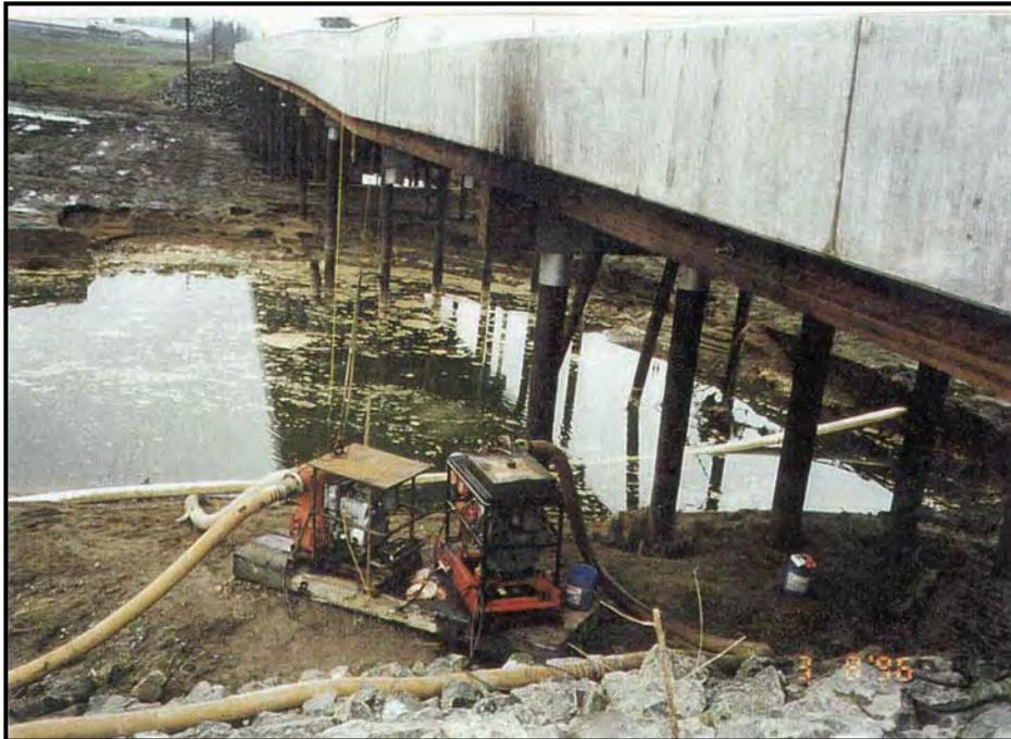
*Figure 6. Looking east along downstream side of Galvin Road overflow bridge into scour hole during dewatering.*
