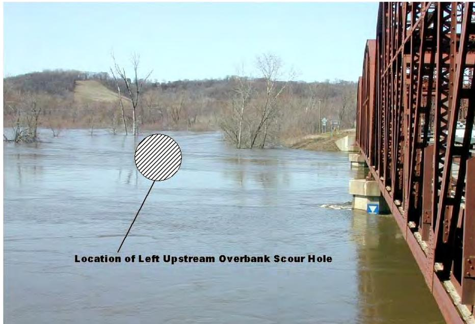
*Figure 5. Looking at flow contraction from left floodplain and location of upstream left overbank scour hole from right upstream abutment of S.R. 25 bridge during April, 2001 flood.*
