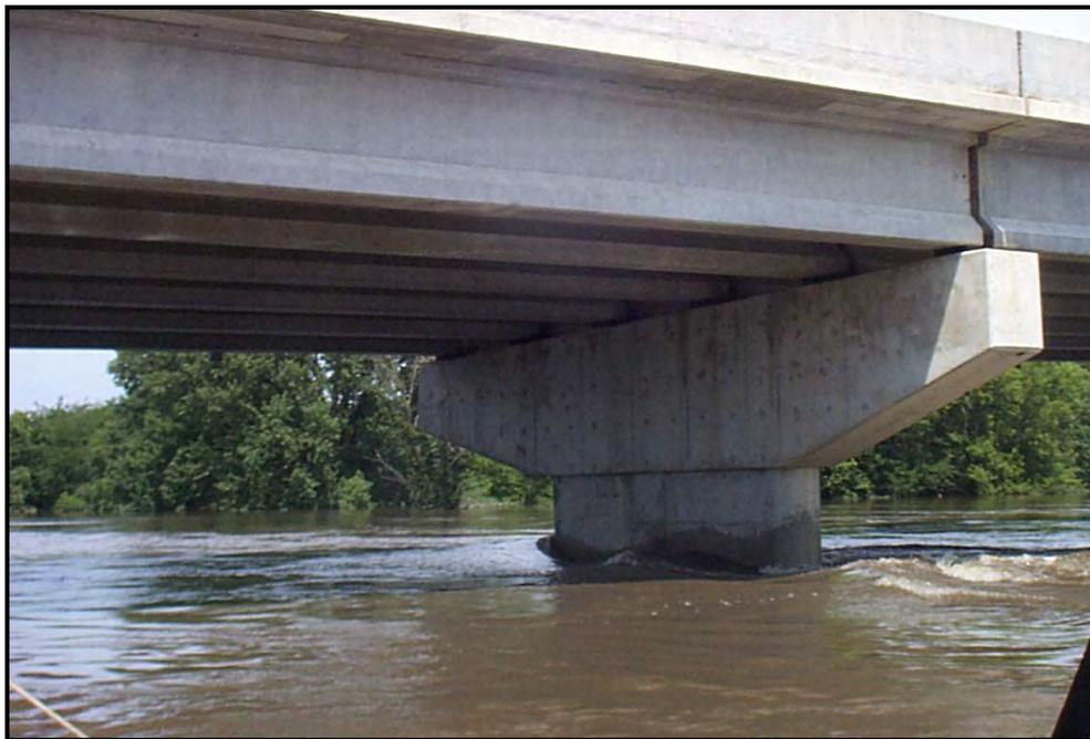
*Figure 6. Looking upstream at wake around Pier 5 of upstream US 218 bridge over the Cedar River, 7/23/1999.*
