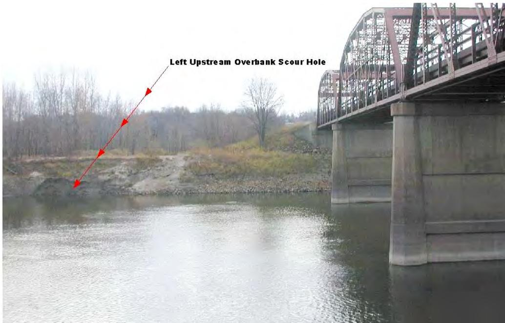
*Figure 6. Looking at left upstream overbank scour hole (inside what appears to have been a much larger scour hole) from right bank along the upstream bridge face of S.R. 25 over the Minnesota River during low-flow.*
