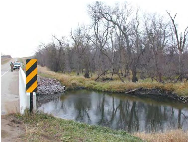
*Figure 6. Looking at scoured area on right upstream bank of County Route 22, during low flow.*
