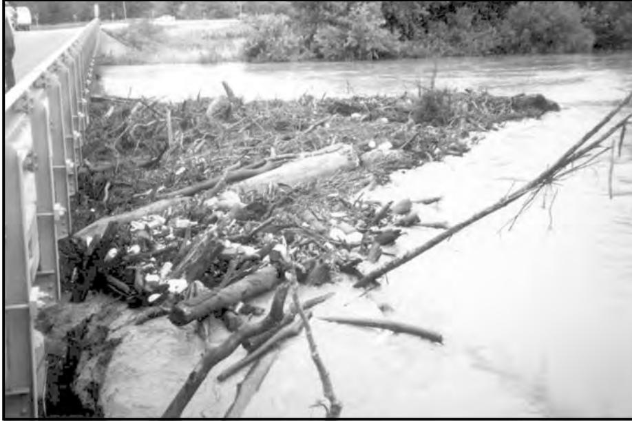
*Figure 9. Looking along upstream S.R. 129 bridge face from left bank at debris raft in front of middle pier (#2) during July 1993 flood.*
