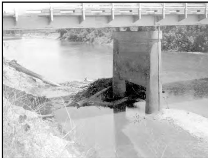
**Figure 6.** Looking upstream at debris raft formed in front of right pier (#3) in June, 1963.
