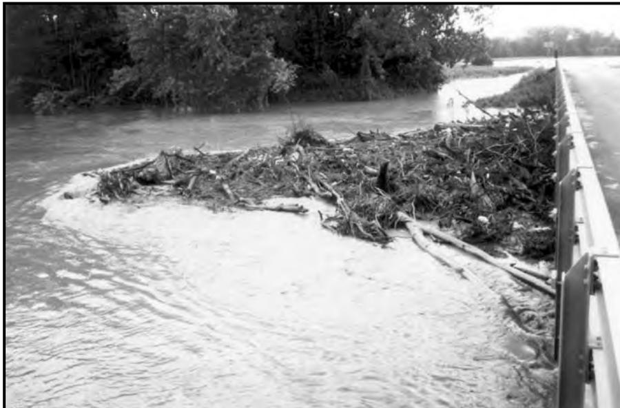
*Figure 8. Looking along upstream S.R. 129 bridge face from right bank at debris raft in front of middle pier (#2) during July 1993 flood.*
