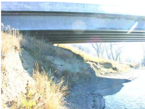
**Figure 8.** Picture of the bank failure at the left abutment of the S.R 37 bridge over the James River near Mitchell, SD taken during low-flow survey following April, 2001 flood.
