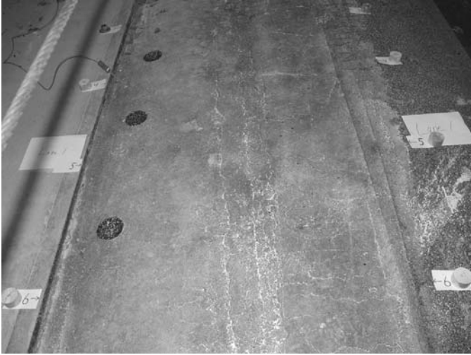
Figure 14. Initial FA-1 test section.
