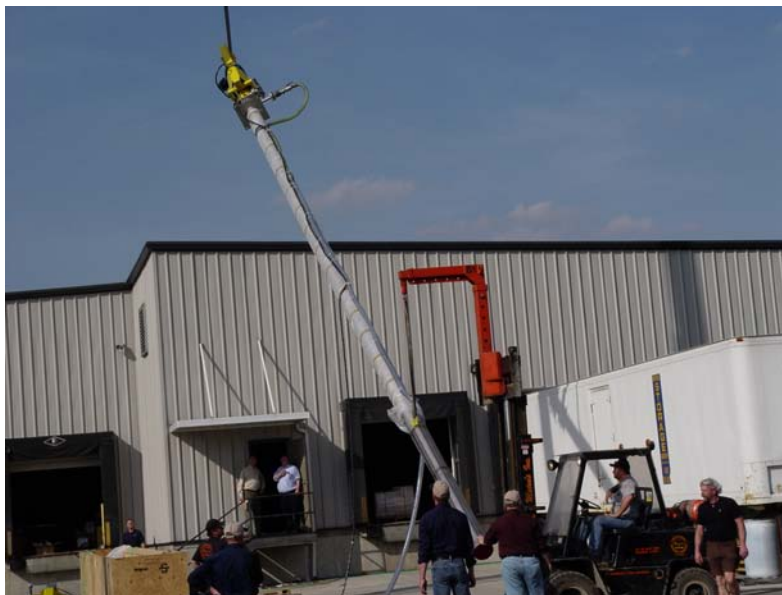
FIGURE III-1 The SEEPEX transfer pump before installation. SOURCE: Reynolds, 2004.
