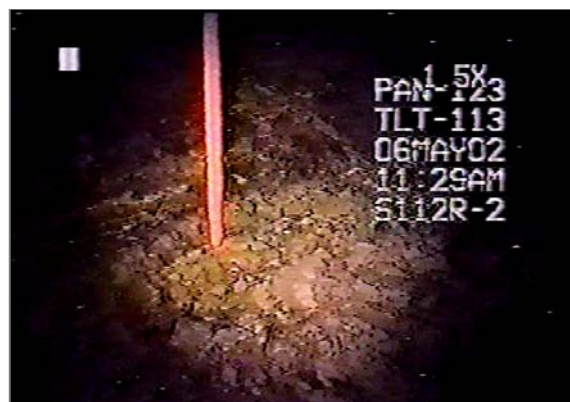
FIGURE G-3 Residual waste on the bottom of Tank S-112 after modified sluicing and saltcake dissolution. SOURCE: Barton, 2005a.
