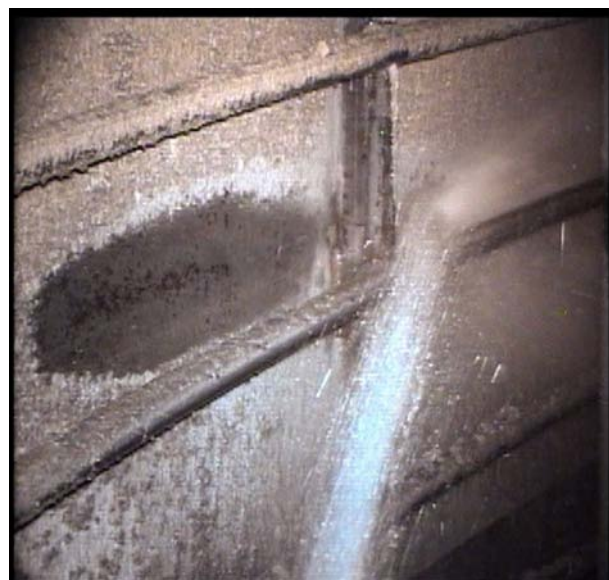
FIGURE G-2 High-pressure water jet used to clean the tank walls at the Idaho site. Note the horizontal cooling coils on the walls. SOURCE: Lockie, 2005b.
