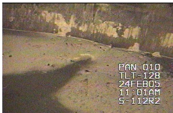
FIGURE G-3 Residual waste on the bottom of Tank S-112 after modified sluicing and saltcake dissolution. SOURCE: Barton, 2005a.
