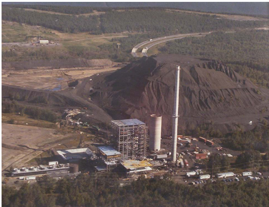
FIGURE 2.6 Westwood FBC plant near Tremont in the southern anthracite field showing a coal refuse pile by the plant.
