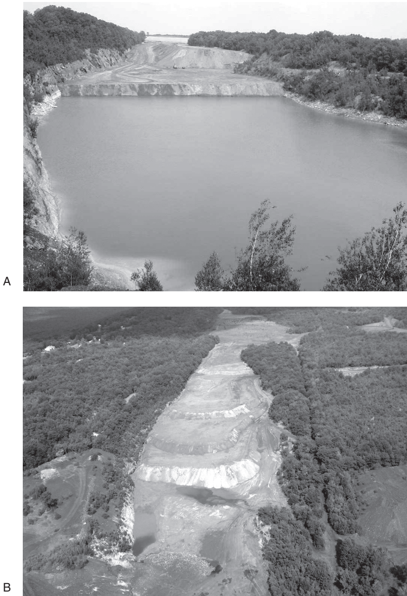
FIGURE 2.8 Big Gorilla pit showing the dry-to-wet placement of approximately three million tons of FBC ash into standing mine water. (A) Big Gorilla in the midst of the placement project. (B) Aerial shot of the filled Big Gorilla pit. NOTE: (A) Courtesy of Barry Scheetz, Pennsylvania State University; (B) Courtesy of Daniel Koury, Pennsylvania Department of Environmental Protection.
