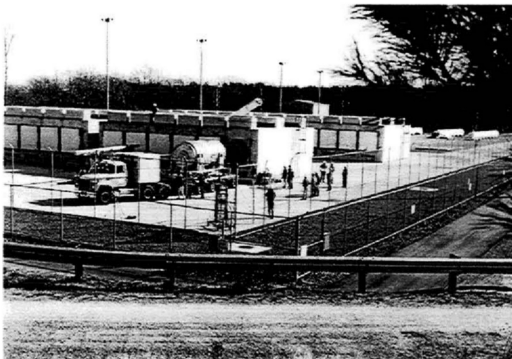
FIGURE 4.2 Photo showing a canister being loaded into a NUHOMS horizontal storage module. SOURCE: Courtesy of Transnuclear, Inc., an Areva Company.
