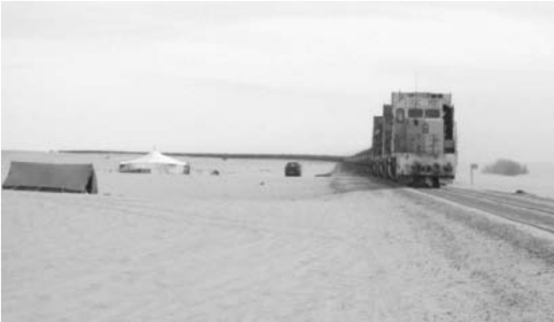
Iron ore railroad operated by the Société Nationale Industrielle et Minière, Mauritania, travels through the Sahara. TTCI engineers performed an onsite study of wheel-rail problems.
