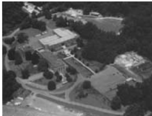
FHWA's Turner-Fairbank Highway Research Center, McLean, Virginia, and demonstration of testing procedure in one of the facility's laboratories. (Photos courtesy of FHWA.)
