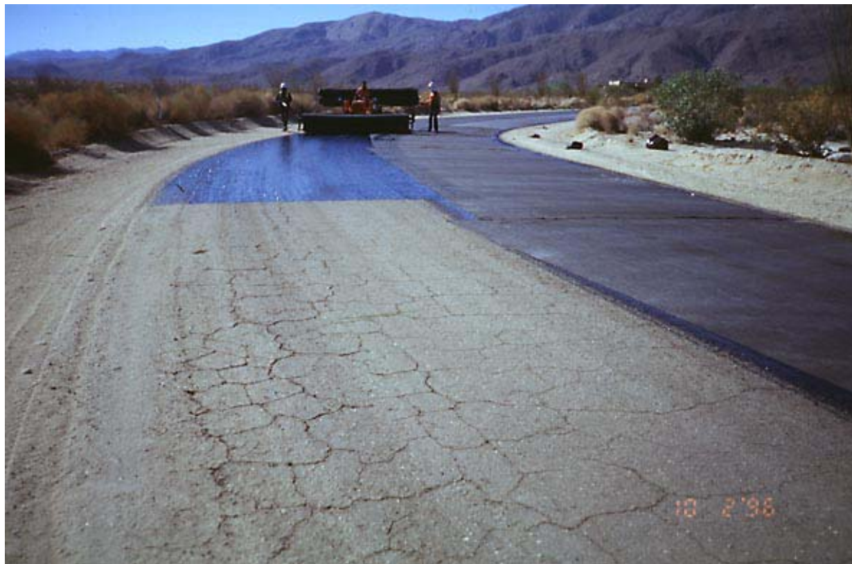
FIGURE 2 Placing fabric has eliminated the need for crack sealing.
