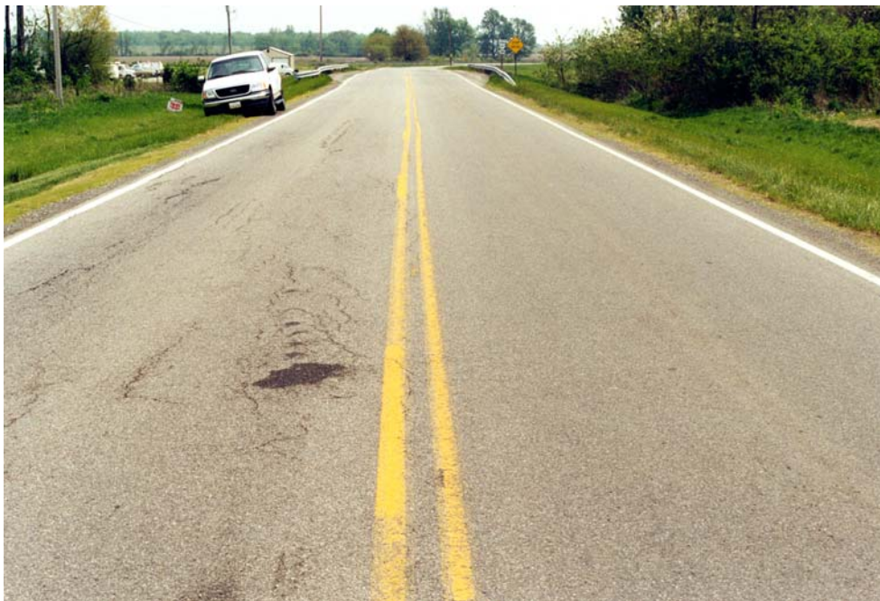
FIGURE 7 Logan County Road 154 in Ohio in July 2002, 5 years after treatment.
