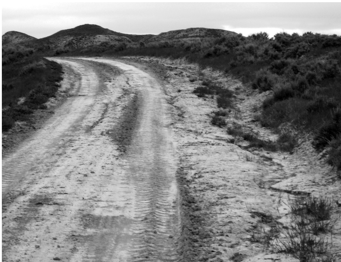
FIGURE 3 County road with small gully in secondary ditch, channeled into main ditch after a recent, heavy rain.
