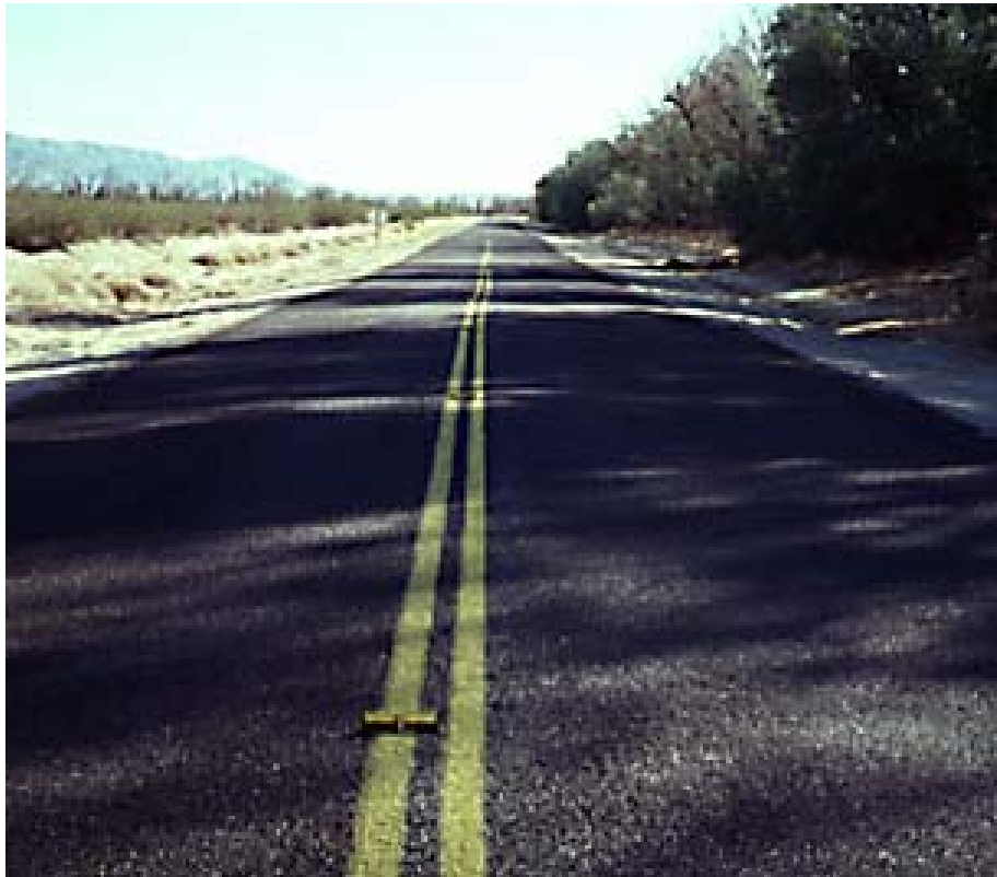
FIGURE 3 Minimum ambient and pavement temperatures, in the sun and shade, must be present before chip sealing begins.
