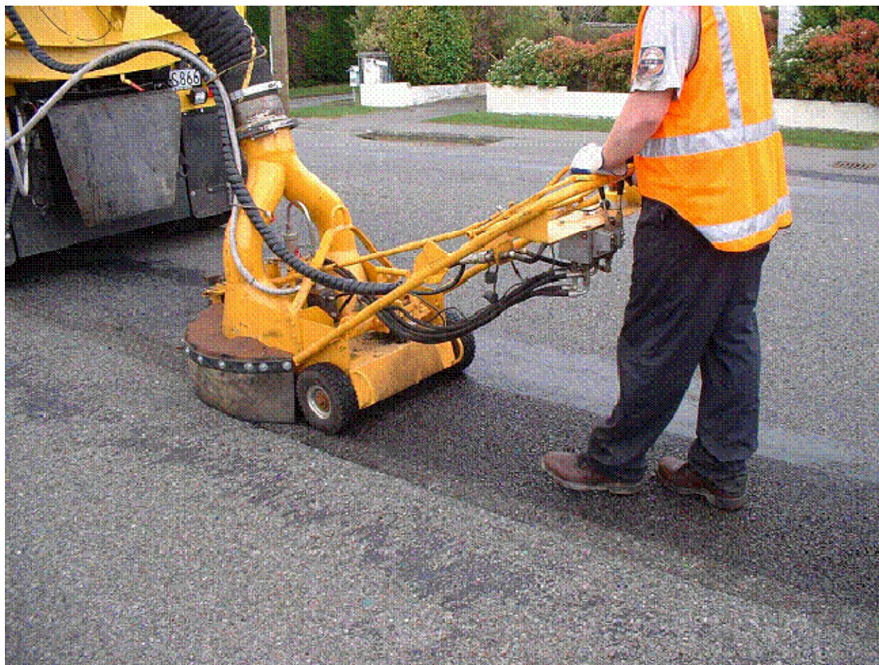
FIGURE 2 Retexturizing using the UHPO watercutter in New Zealand (15).
