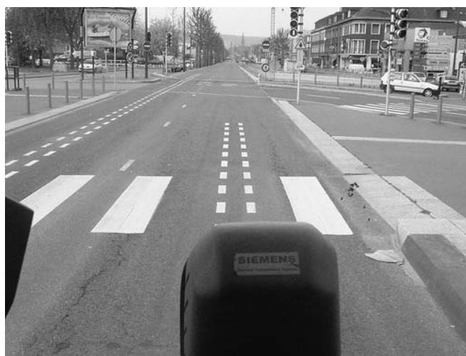
Figure 9 Special street lines that are part of Rouen's automatic bus guidance system.
